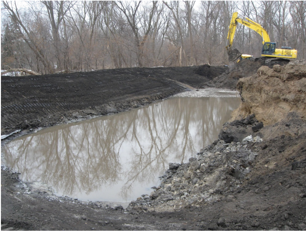
Continuing excavation of the basin
