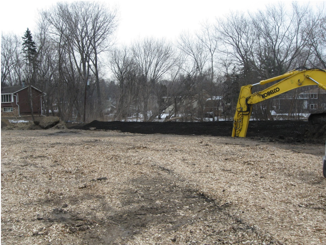
Starting excavation of the basin
