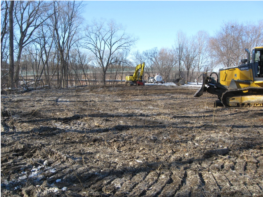
Nature area after clearing and grubbing
