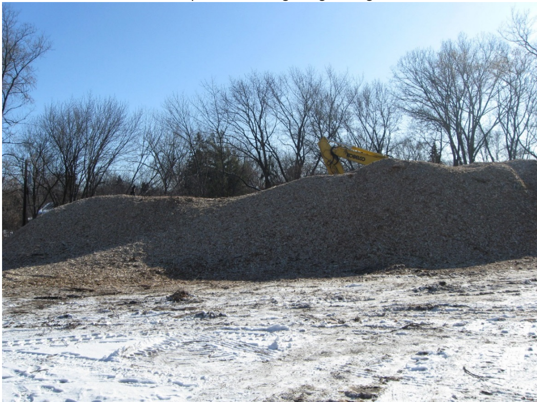
Wood chips from clearing and grubbing
