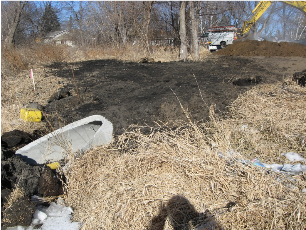
Installation of outlet pipe to Bassett Creek
