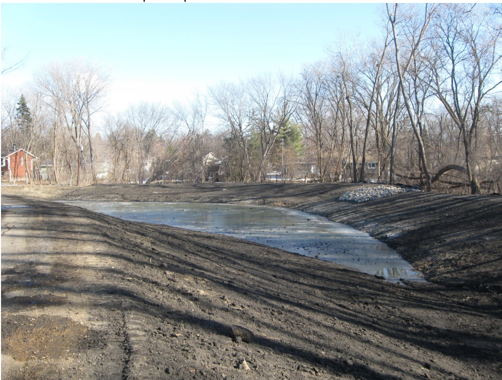
Completed pond basin
