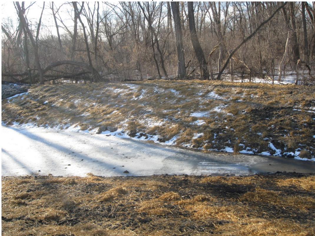
Basin with temporary stabilization
