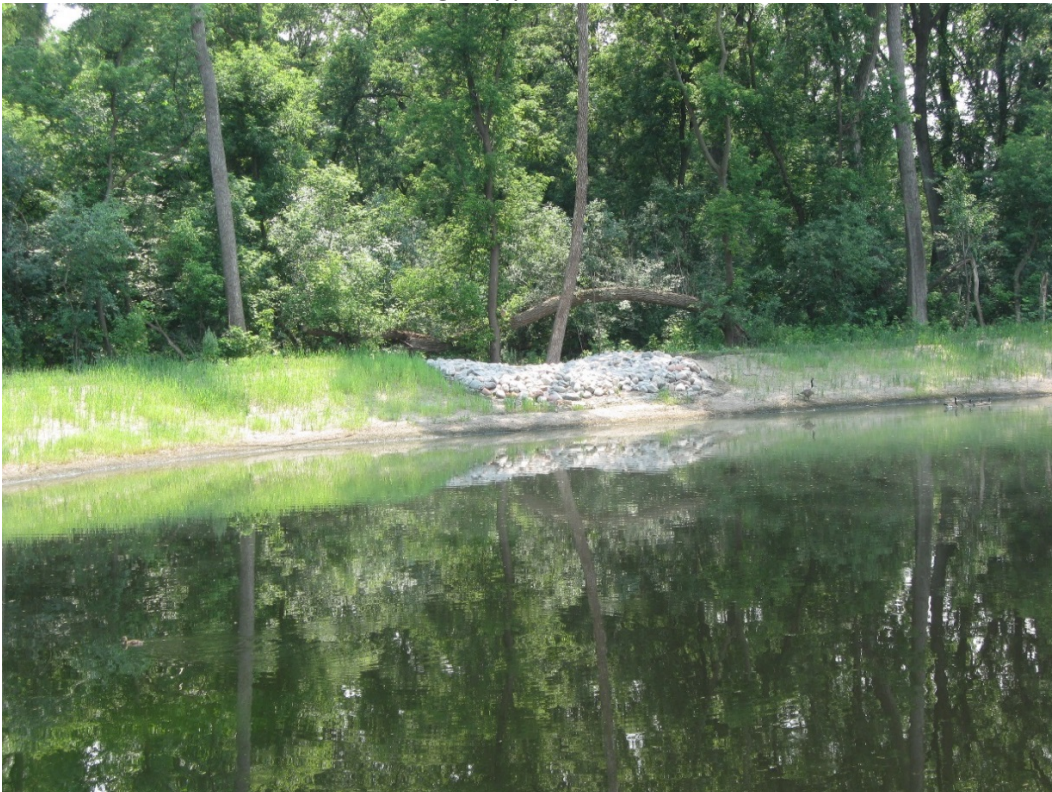
Emergency pond overflow
