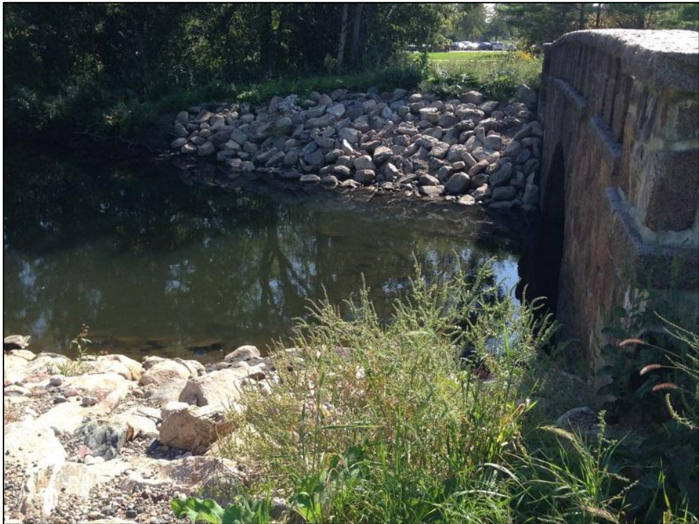
Site 4 – Parkway Bridge – 127+50 – AFTER
