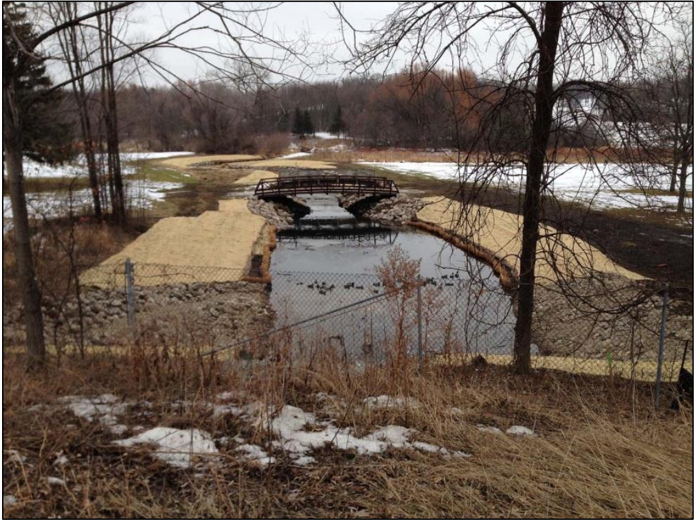
Sites 7 and 7a – Golden Valley Road – DURING CONSTRUCTION
