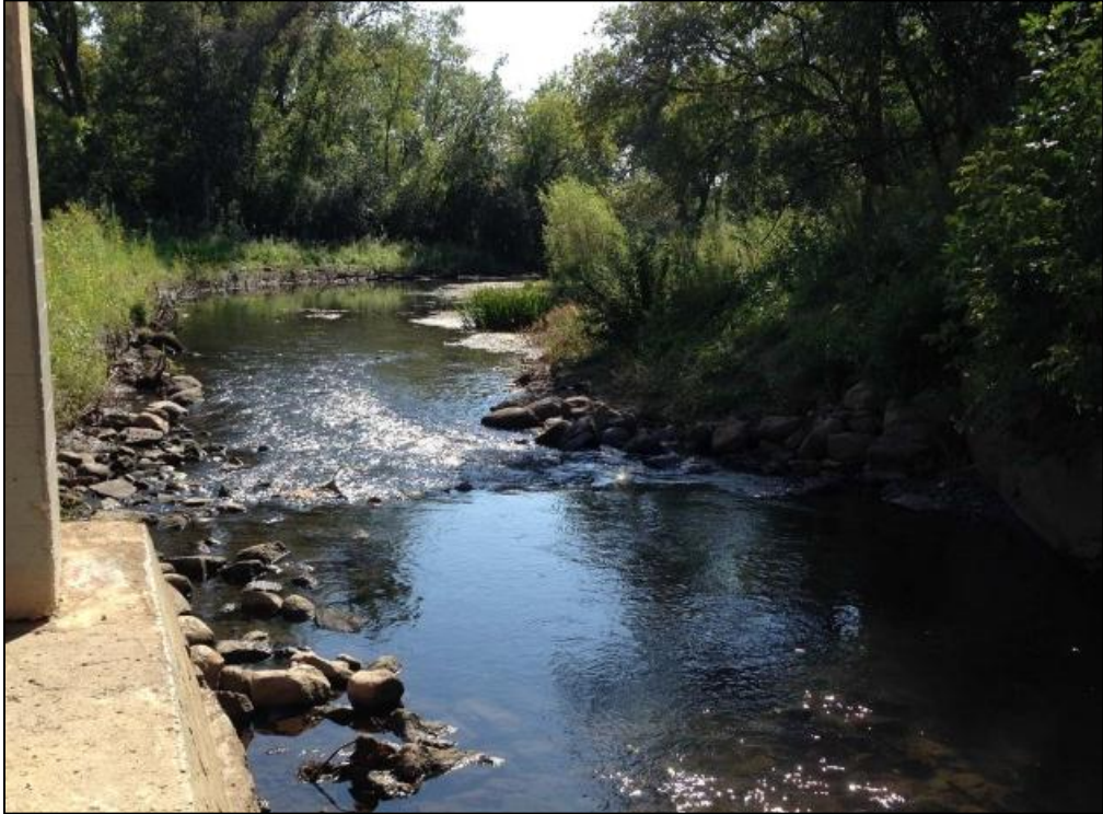
Site 4 – Parkway Bridge – 127+50 – AFTER
