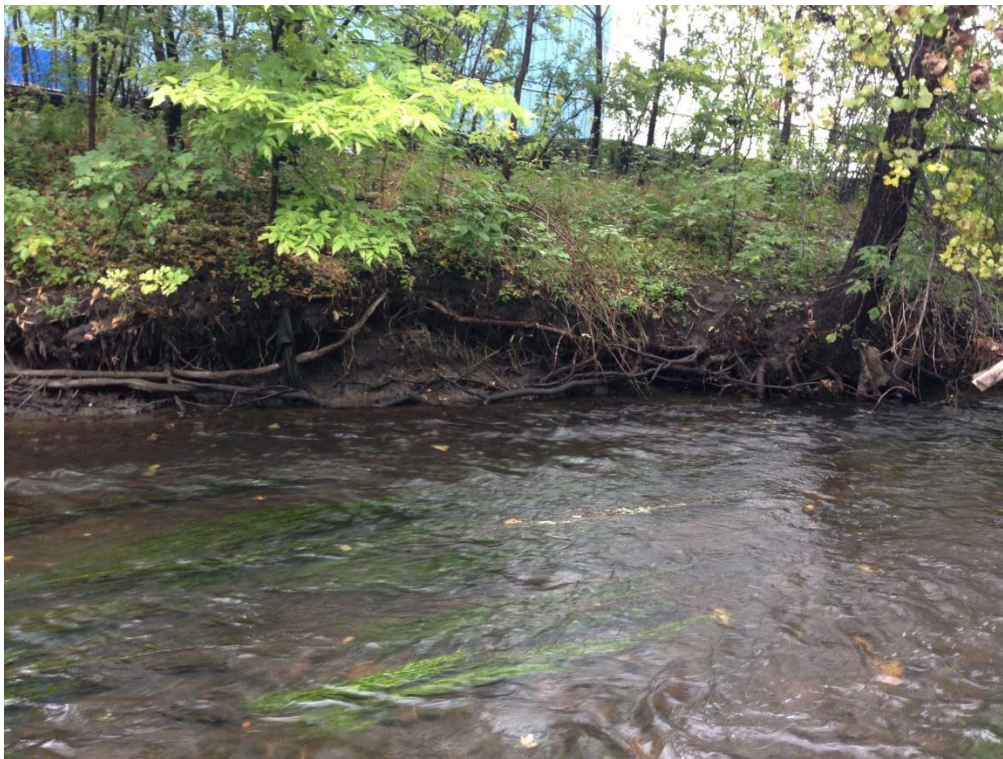
Photo 12. Site 12. Minor to moderate erosion on stream bank downstream of riprap
