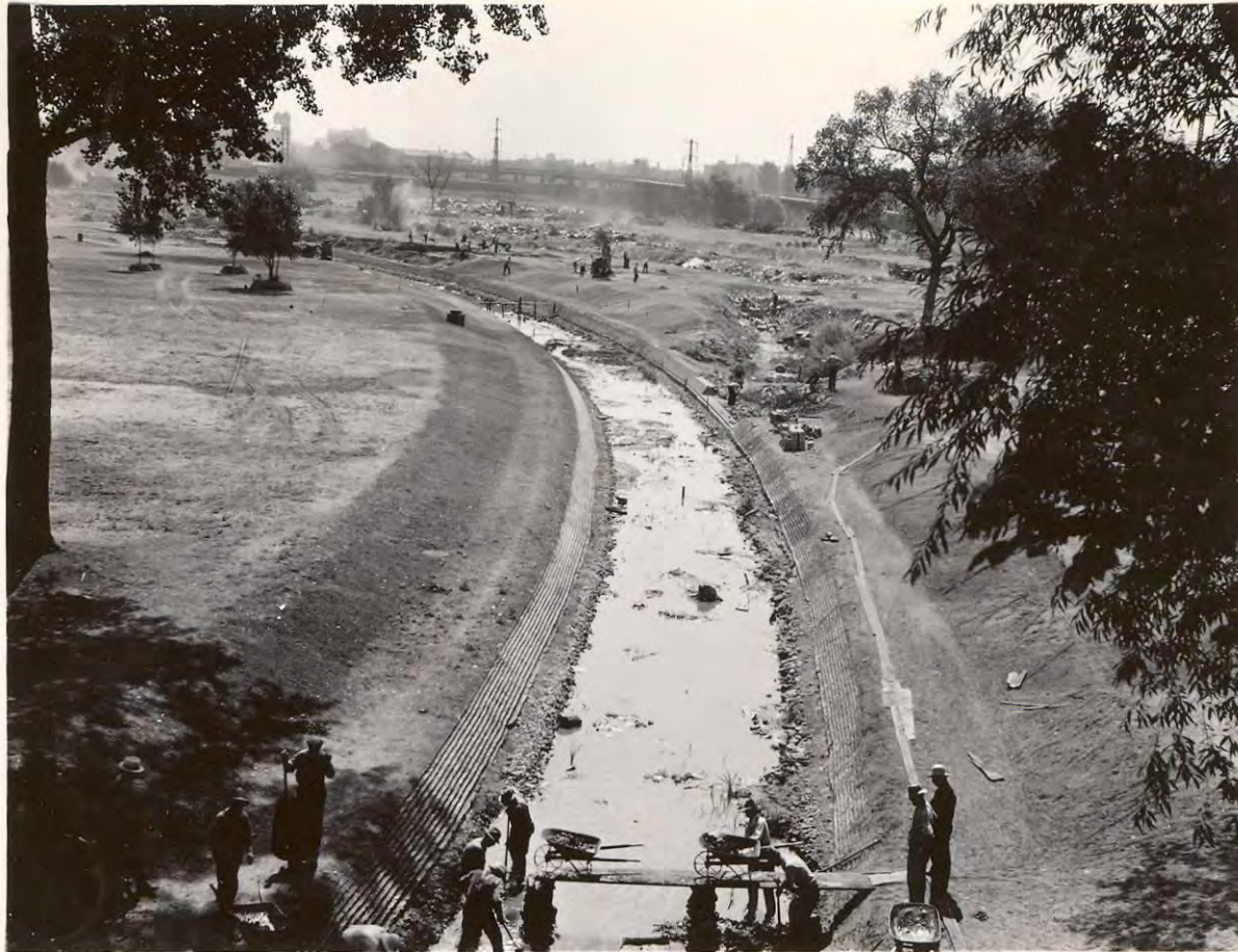
Riprapping Bassett's Creek and clearing channel.
