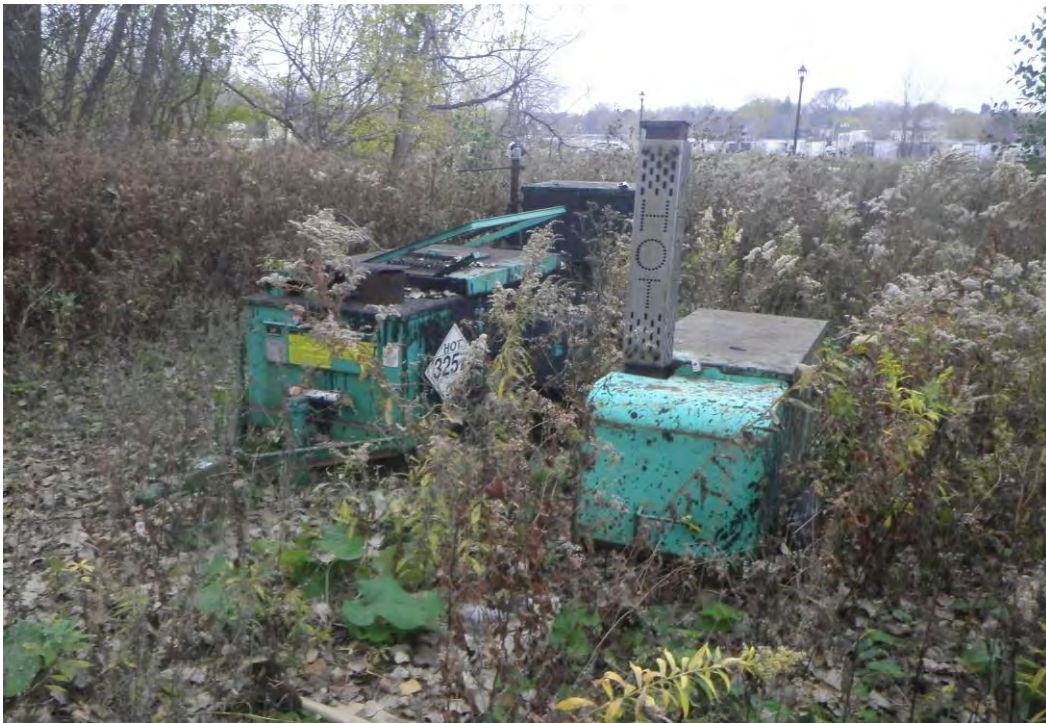
Photo 10: Abandoned equipment and material storage
