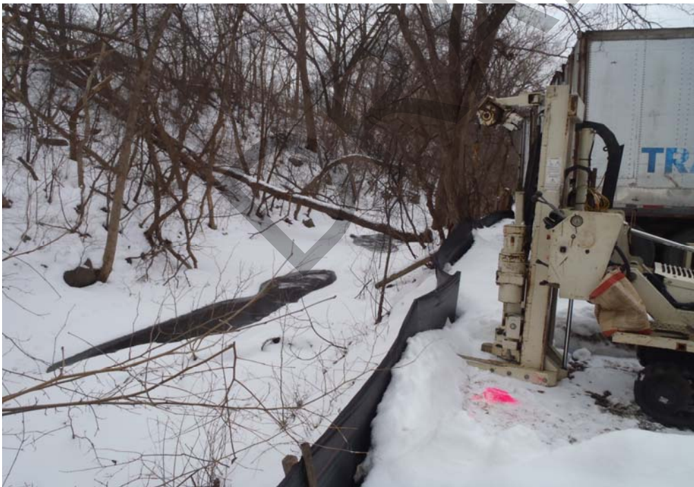
Photo 7: Geoprobe Setup at SB-15-05
