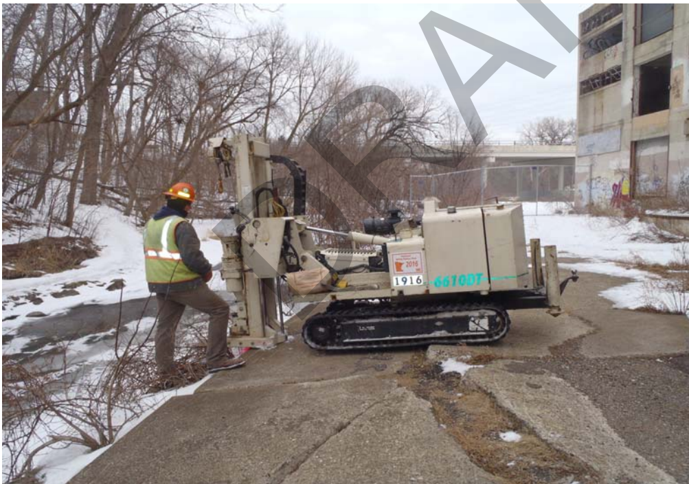
Photo 1: Geoprobe Setup at SB-15-01
