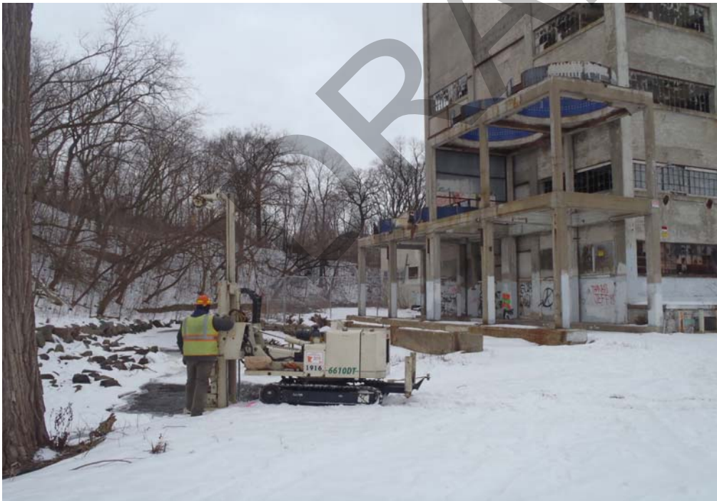
Photo 3: Geoprobe Setup at SB-15-02
