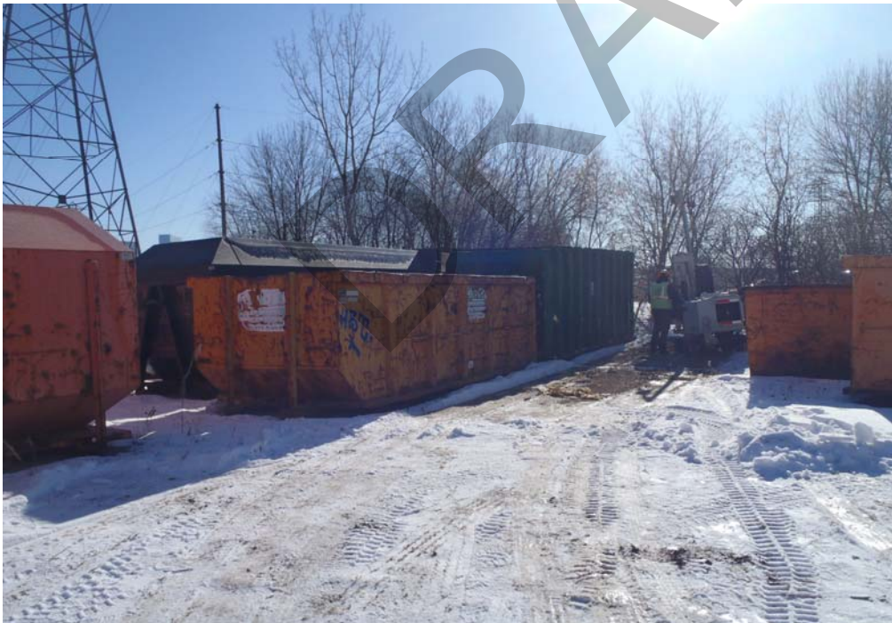
Photo 13: Geoprobe Setup at SB-15-08
