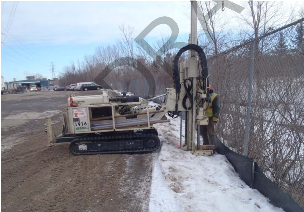
Photo 9: Geoprobe Setup at SB-15-06
