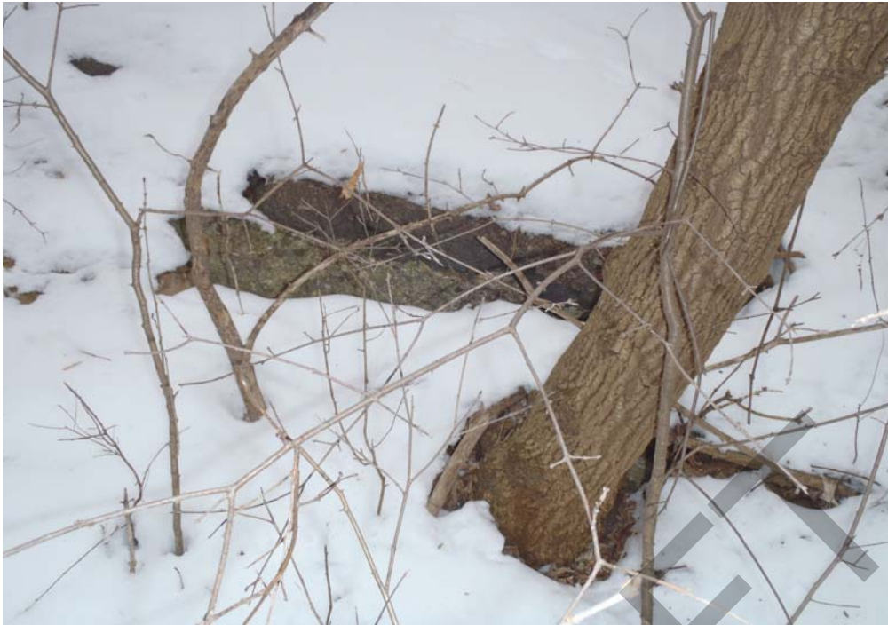
Photo 16: Debris Around SP-15-09 (Concrete and Blacktop)
