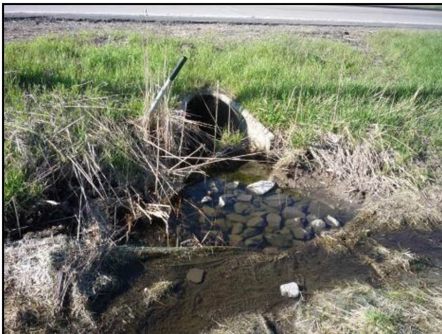
Figure 3.3. 24 inch reinforced concrete pipe. Pipe leads flow from ditch to Four Seasons Mall delineated wetland area.
