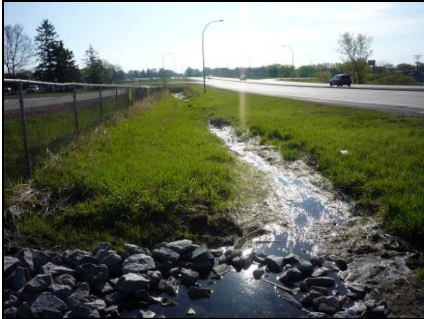
Figure 3.2. Rockford Road roadside ditch. Facing east from storm sewer outlet toward the connecting culvert directing flow towards the Four Seasons Mall.
