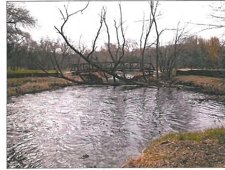
LOOKING SOUTH DOWNSTREAM
