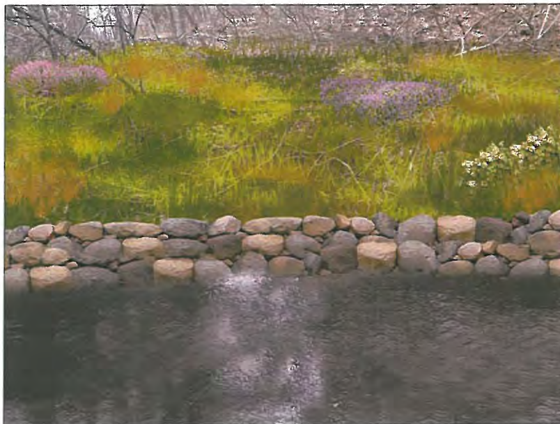
INSTALL BOULDER TOE STABILIZATION
