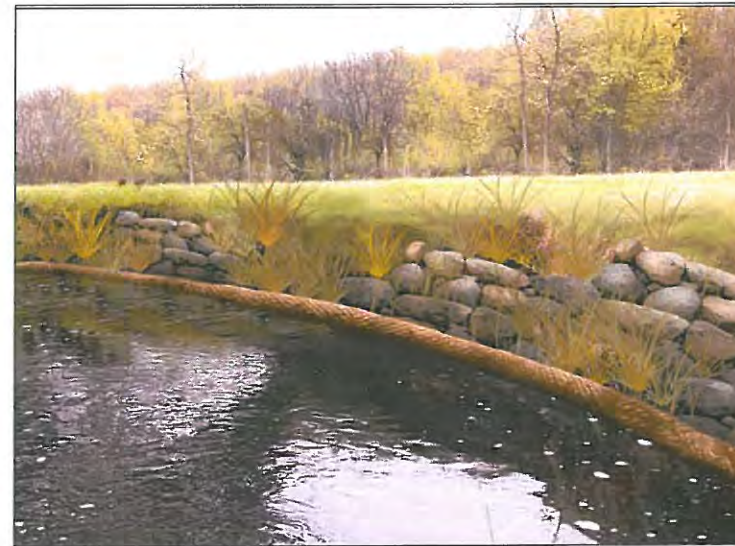
RESHAPE SLOPE AND INSTALL TREE REVETMENT
