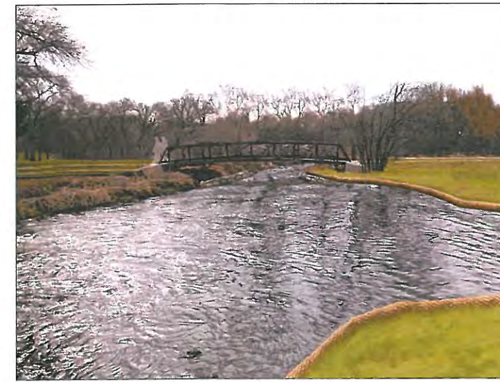
RESHAPE SLOPE AND INSTALL BIO-LOG
