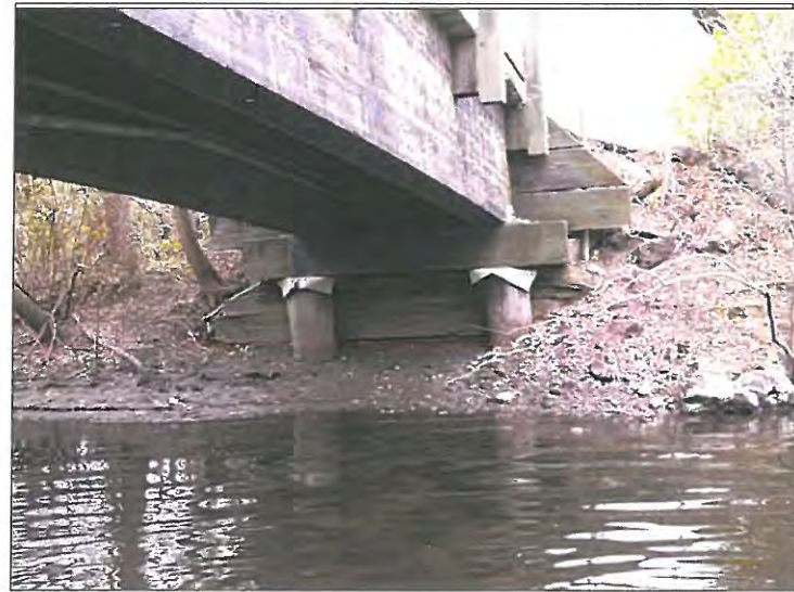
LOOKING EAST UNDER THE BRIDGE
