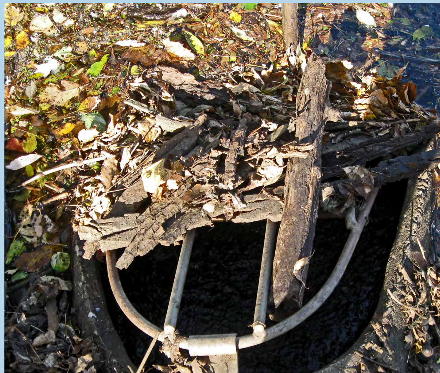
Downed trees and exposed soils in channel, debris blocking outlet, and accumulated sediment at storm sewer outfall to DeCola Pond B
