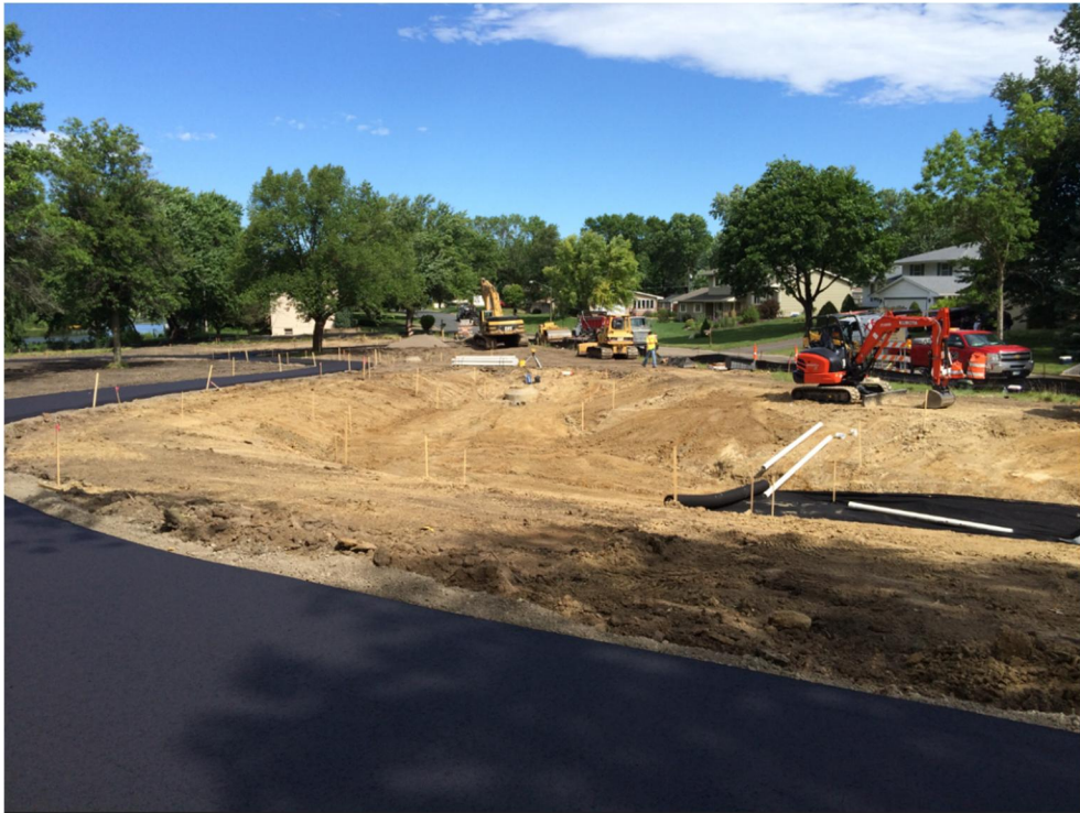
Rain Garden Construction
