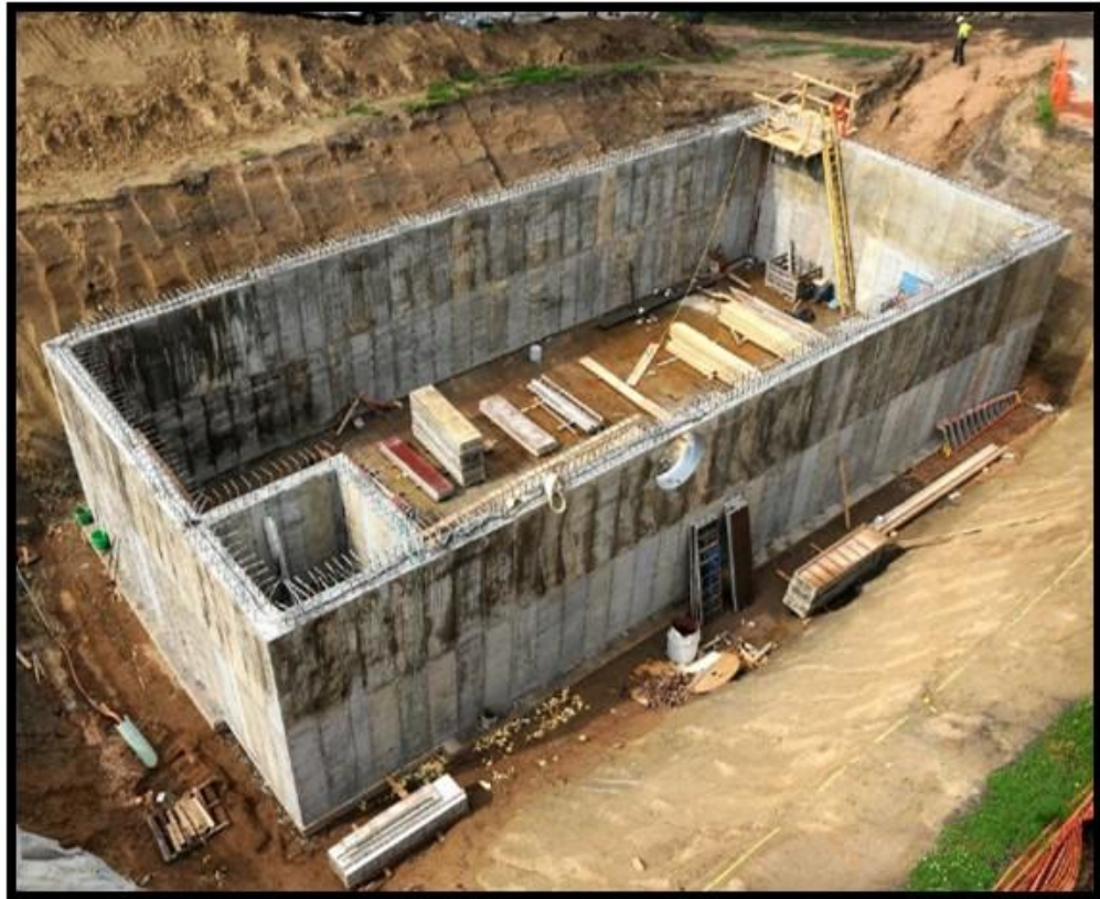
Underground Storm Water Reuse Tank
