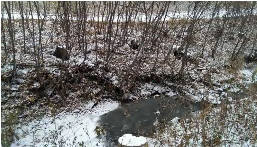
Figure 38 – Parkers Lake, Reach 2, bank scarp erosion
