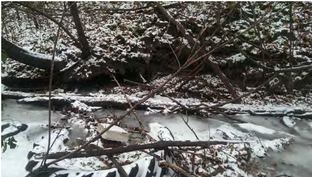
Figure 15 – Mt. Olivet, Reach 3, bank scarp erosion caused by debris in channel
