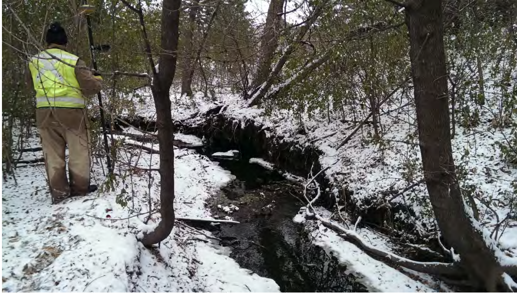
Figure 23 – Parkers Lake, Reach 1 bank scarp erosion
