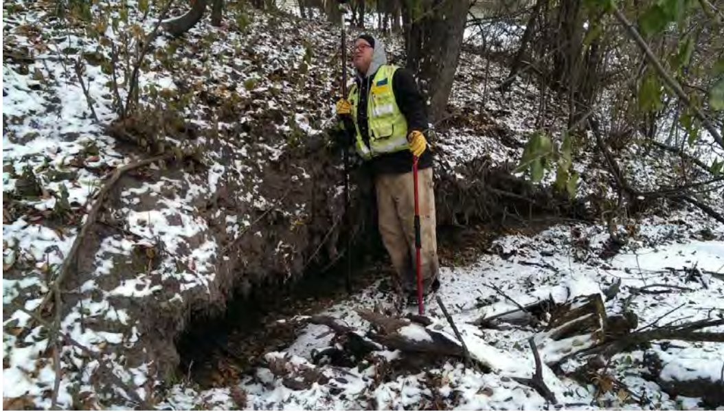
Figure 9 – Mt. Olivet, Reach 2, undercut bank and bank erosion cause by debris in channel
