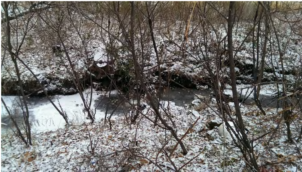
Figure 42 – Parkers Lake, Reach 2, undercut bank and bank erosion
