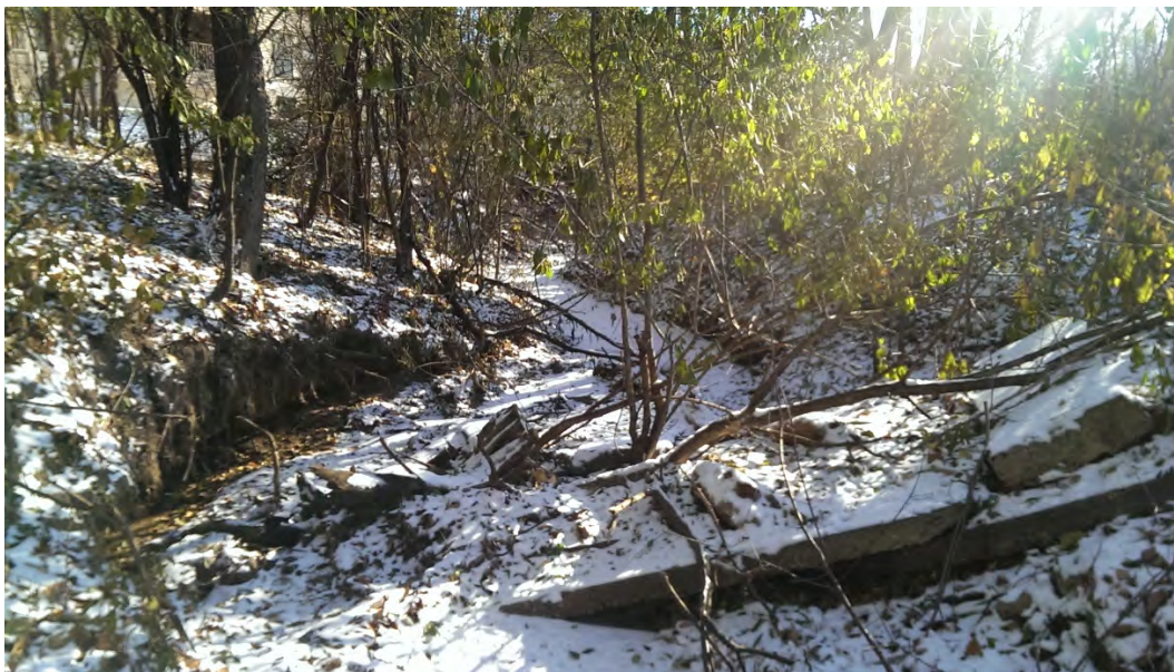
Figure 4 – Mt. Olivet, Reach 2, undercut bank and bank erosion cause by debris in stream channel
