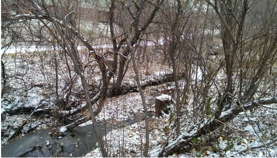
Figure 39 – Parkers Lake, Reach 2, bank erosion
