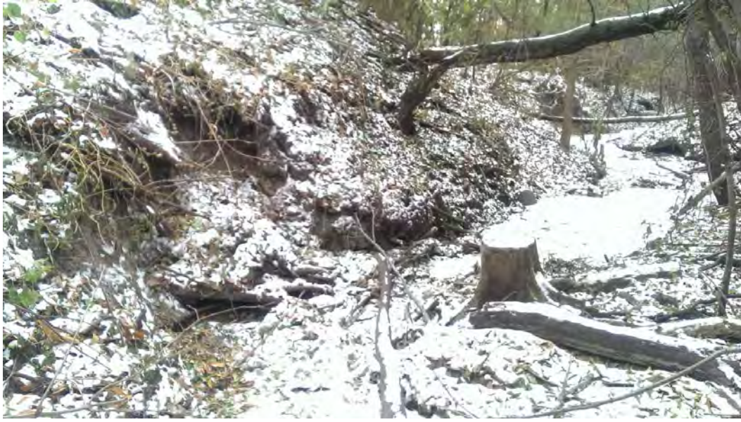
Figure 16 – Mt. Olivet, Reach 3, bank scarp erosion
