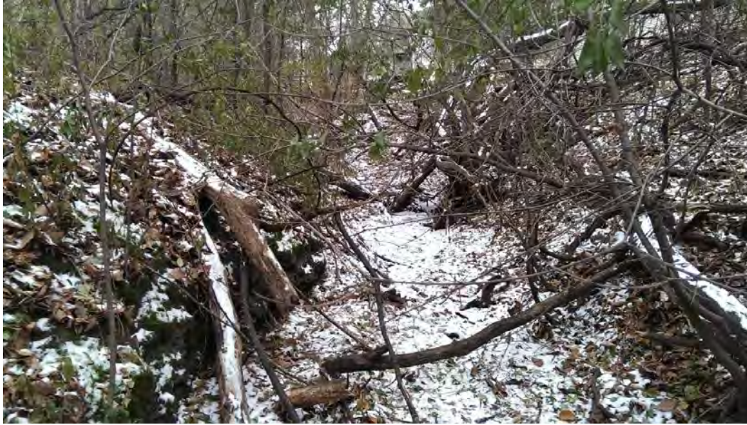
Figure 3 – Mt. Olivet, Reach 2, bank scarp erosion
