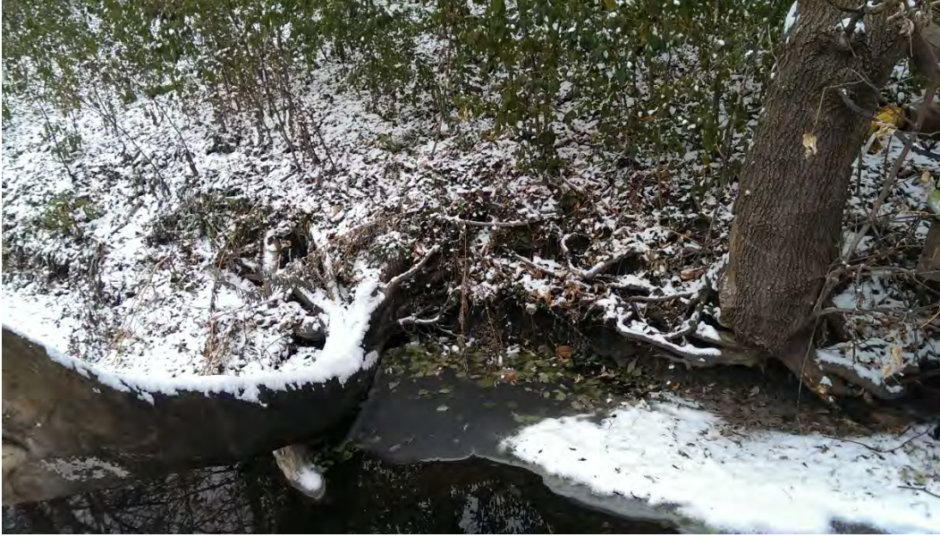
Figure 27 – Parkers Lake, Reach 1, undercut bank (zoomed in of previous figure)
