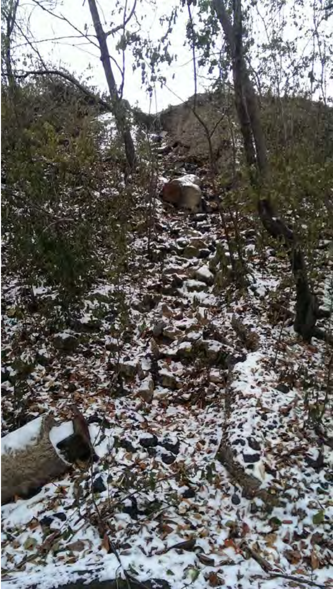
Figure 13 – Mt. Olivet, Reach 2, slope erosion from parking lot down to the stream (view from below, same location as previous two figures)
