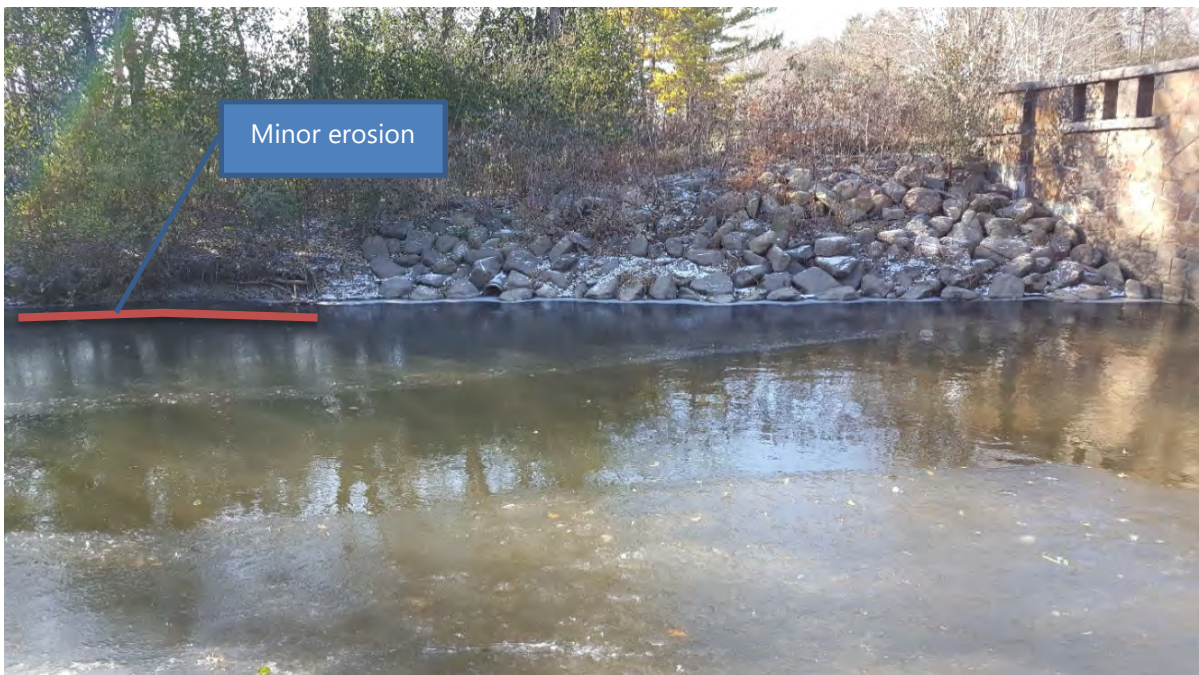
Figure 3-5 Erosion within right overbank of the channel downstream of the riprap (upstream of Lagoon E)
