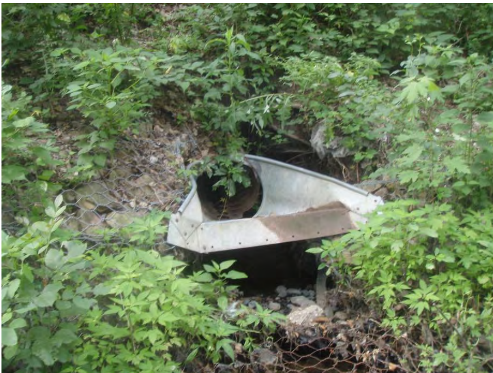
Photo 14. Site 9. Erosion around flared end section.
