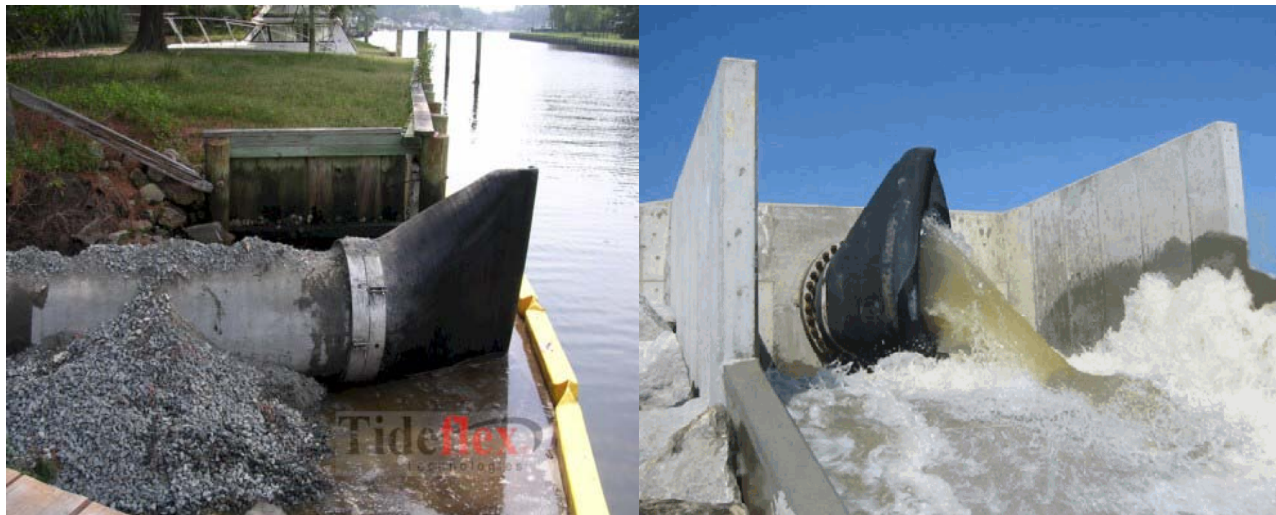
Figure 4. Photos of the Rubber Check Valve.
