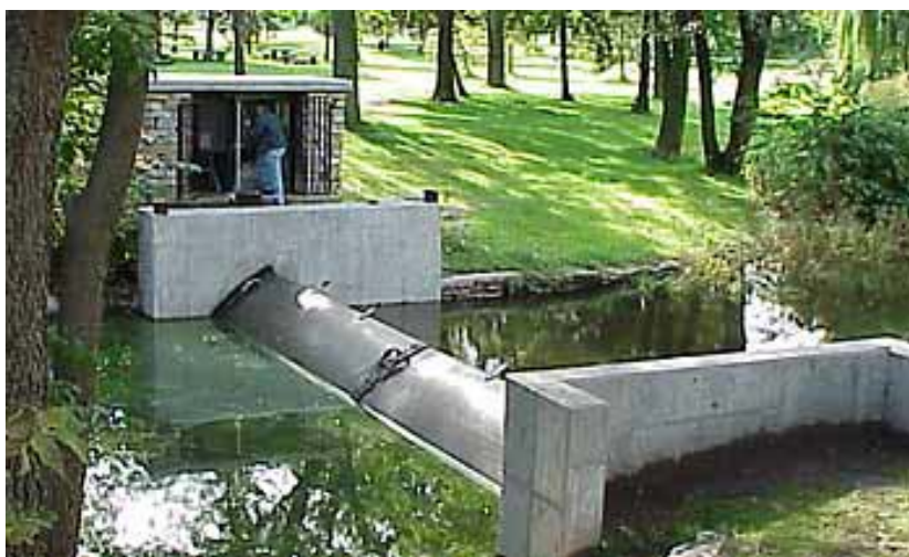
Figure 5. Inflatable barrier at Minnehaha Creek and Lake Nokomis.
