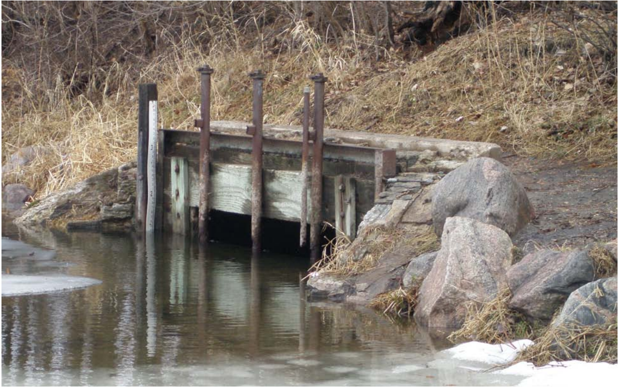
Figure 2. Existing Wirth Lake Outlet Structure.
