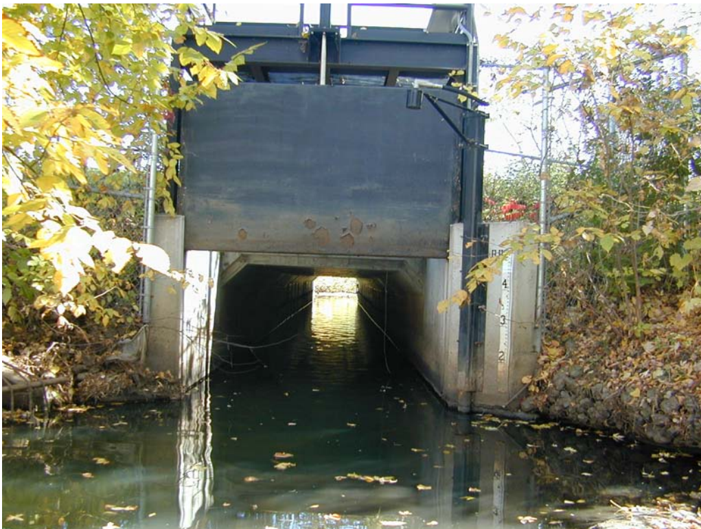
Figure 3. Example of an automated steel lift gate at Wisconsin Avenue in the City of Golden Valley.
