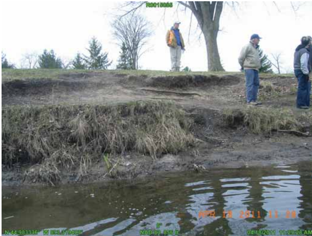
Photo 4. Site 2. Severely eroding bank near box culvert entrance
