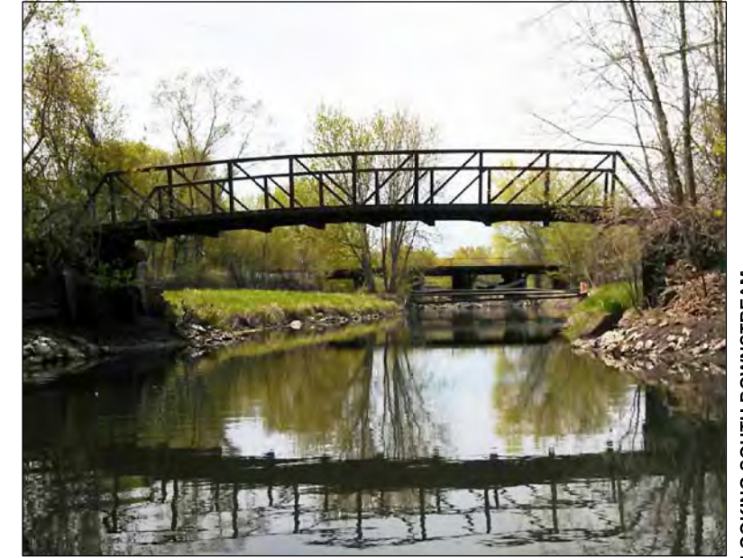
LOOKING SOUTH DOWNSTREAM
