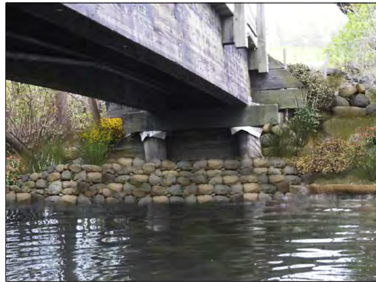
INSTALL BOULDER TOE
