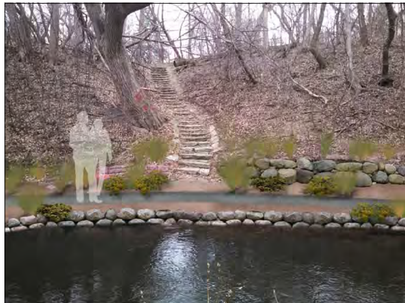
INSTALL BOULDER TOE STABILIZATION REPLACE WODDEN RETAINING WALL AND REESTABLISH TRAIL
