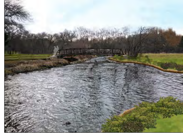
RESHAPE SLOPE AND INSTALL BIO-LOG
