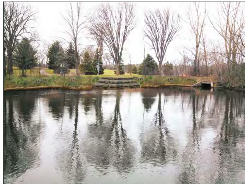
RESHAPE SLOPE AND INSTALL STONE STAIRS
