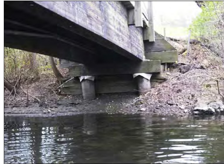
LOOKING EAST UNDER THE BRIDGE
