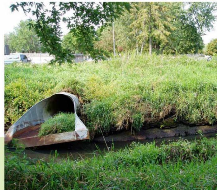
Erosion is frequently observed at culvert outlets for a variety of reasons, including insufficient erosion protection at the culvert outlet, streambank erosion, and channel downcutting, which leaves the culvert perched above the channel. Filter fabric is often used at culvert outlets to separate riprap protection from underlying soils, however the fabric provides a slippery surface for the riprap, which commonly slides into the channel.
