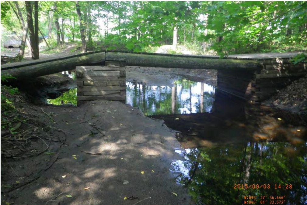
Photo 6. Site 6. Erosion around bridge abutments
