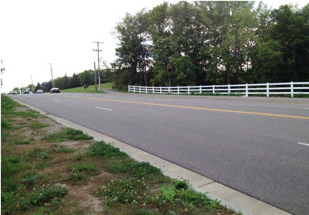
Photo 11: Fernbrook Lane, looking north
