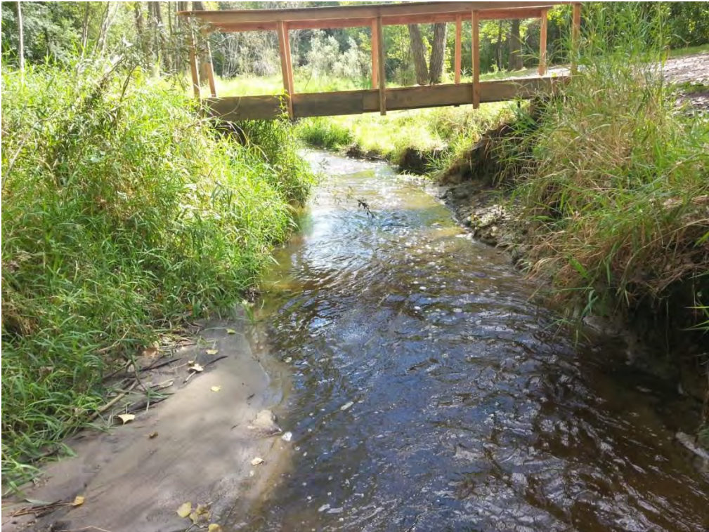
Photo 8. Site 9. Erosion around bridge abutments
