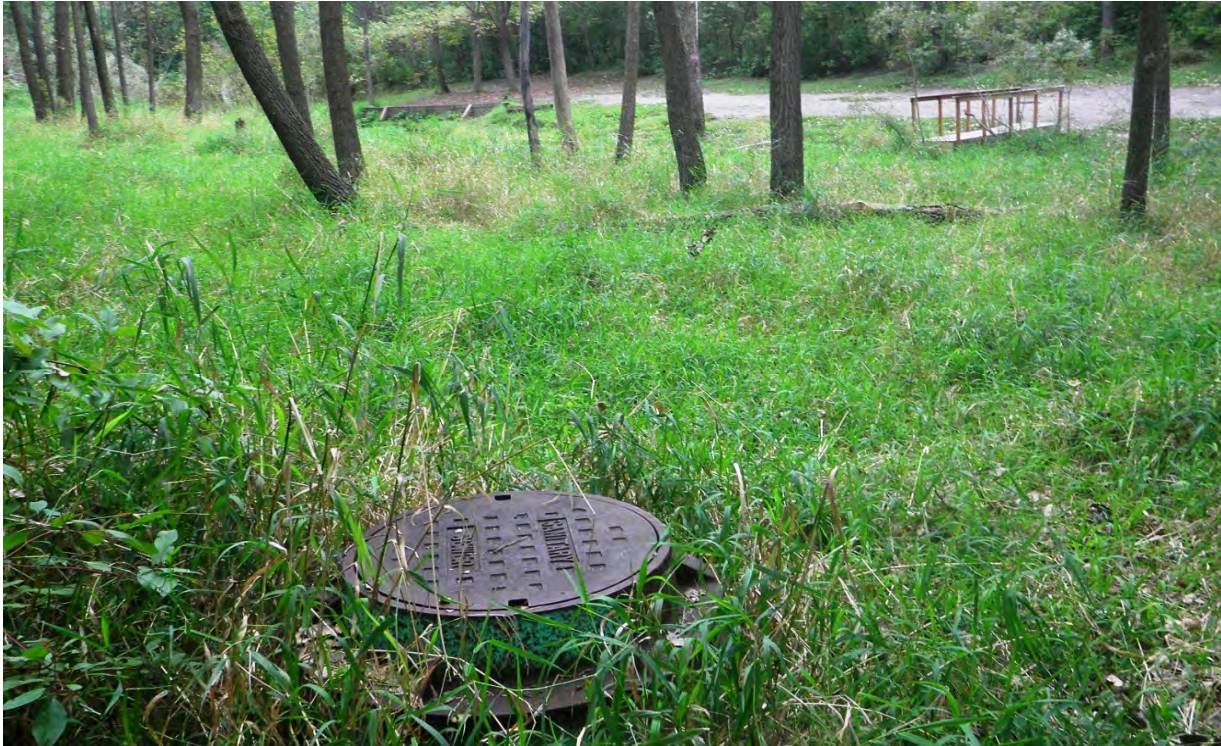
Photo 9: Sanitary sewer manhole, creek in background
