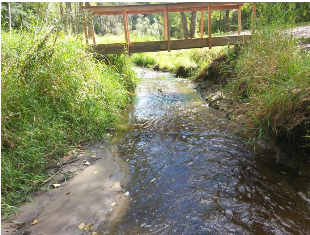
Photo 8. Site 9. Erosion around bridge abutments
