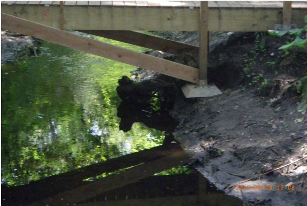
Photo 8. Site 9. Erosion around bridge abutments
