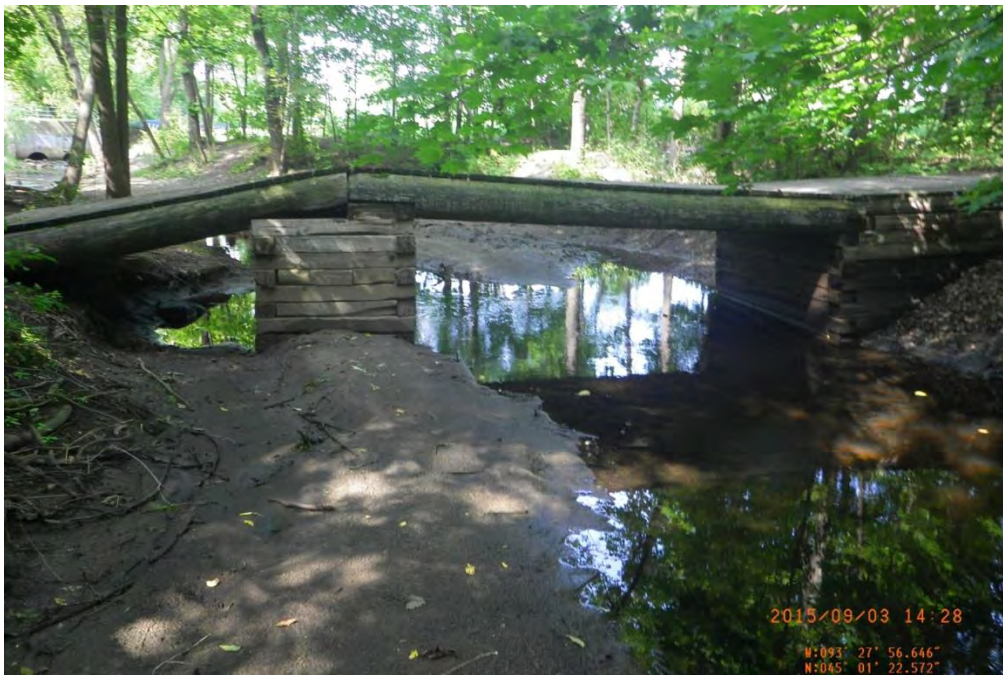
Photo 6. Site 6. Erosion around bridge abutments
