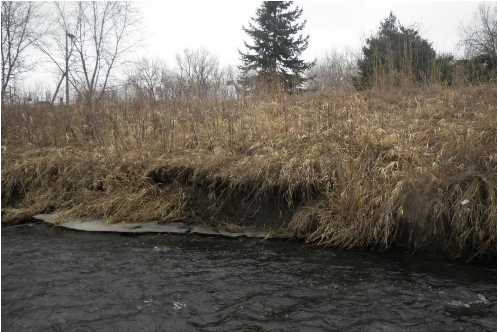
Photo 9. Site 9. Undercut bank
