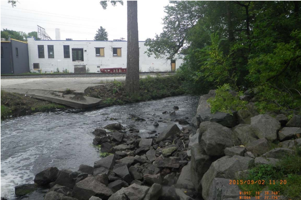
Photo 4. Site 4. Undercut swale and downstream bank
