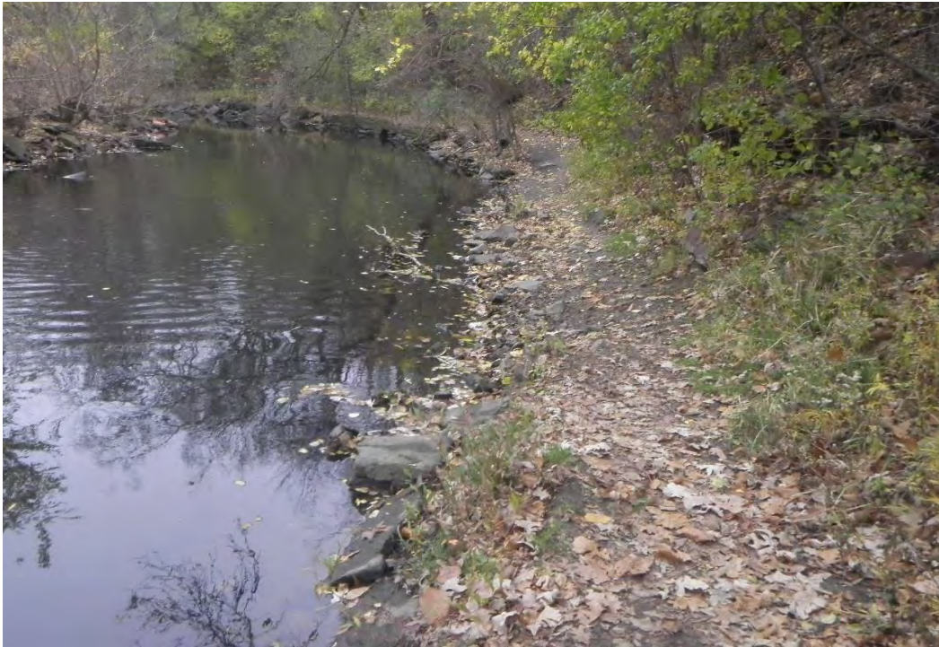
Photo 1: Fruen Mill Reach Stabilization Area 1, looking east
