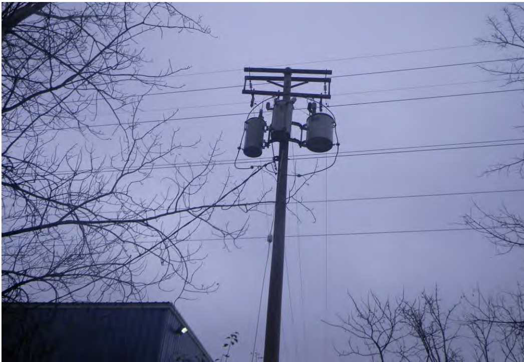
Photo 12: Pole-mounted transformer
