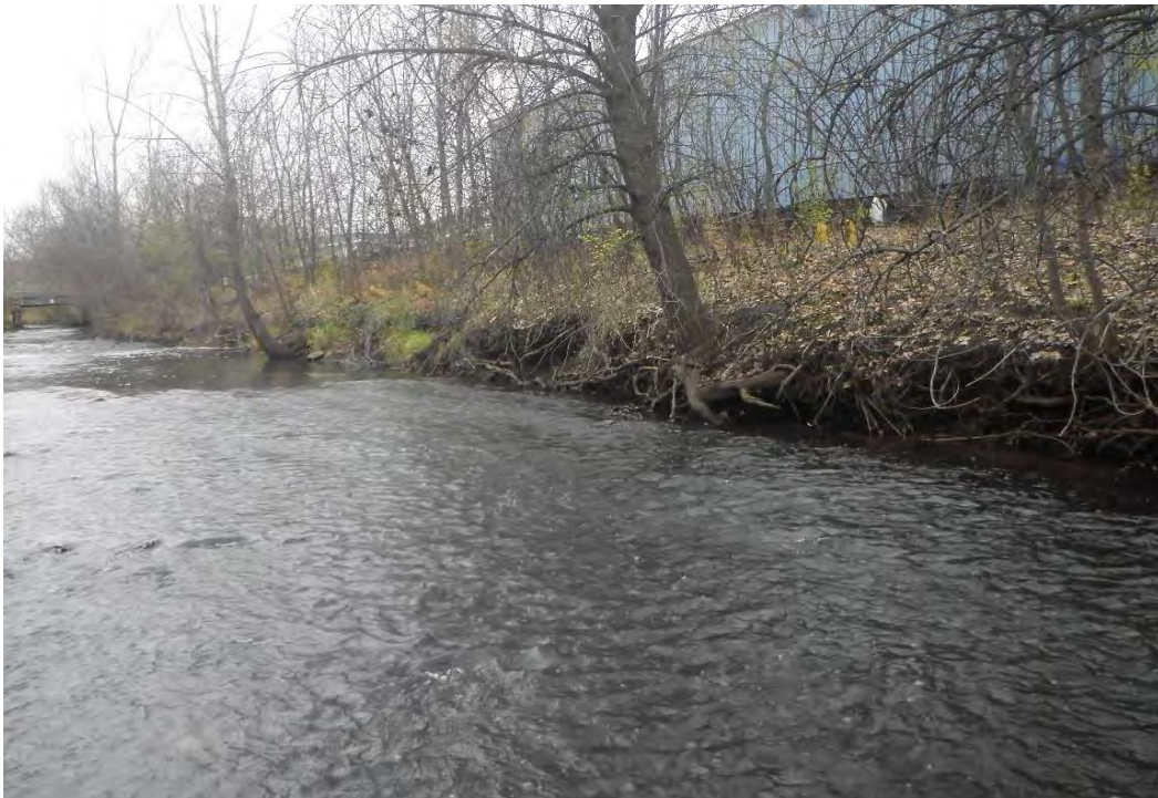
Photo 6: Dupont/2nd Ave Reach Stabilization Area 6
