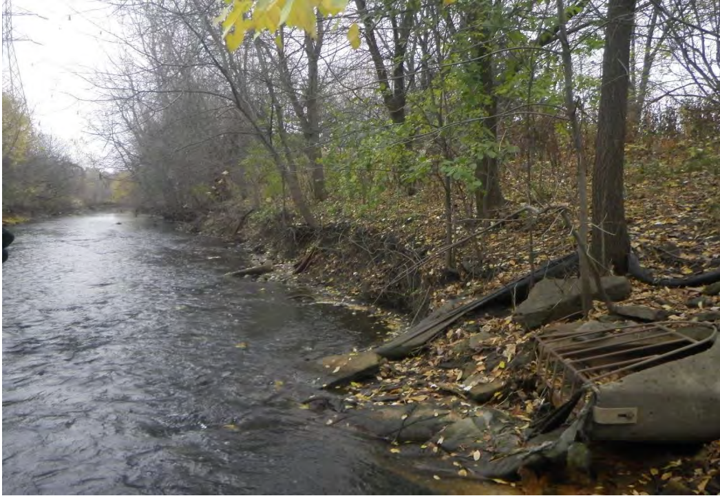
Photo 7: Dupont/2nd Ave Reach Stabilization Area 7
