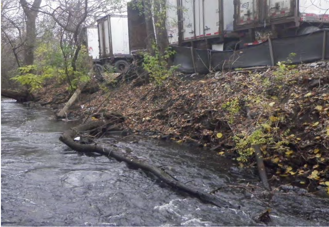
Photo 5: Cedar Lake Reach Stabilization Area 5
