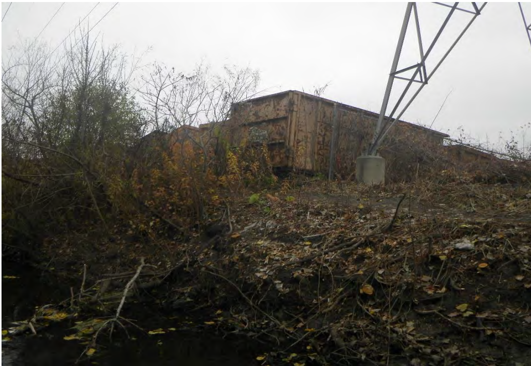
Photo 8: Dupont/2nd Ave Reach Stabilization Area 8
