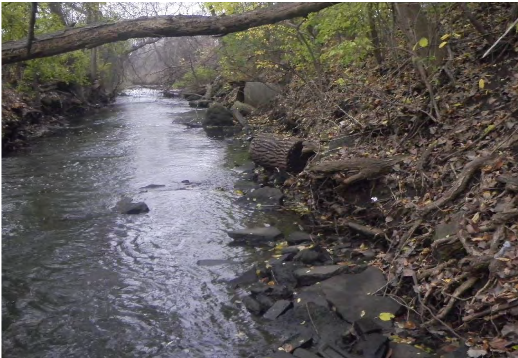
Photo 4: Cedar Lake Reach Stabilization Area 4
