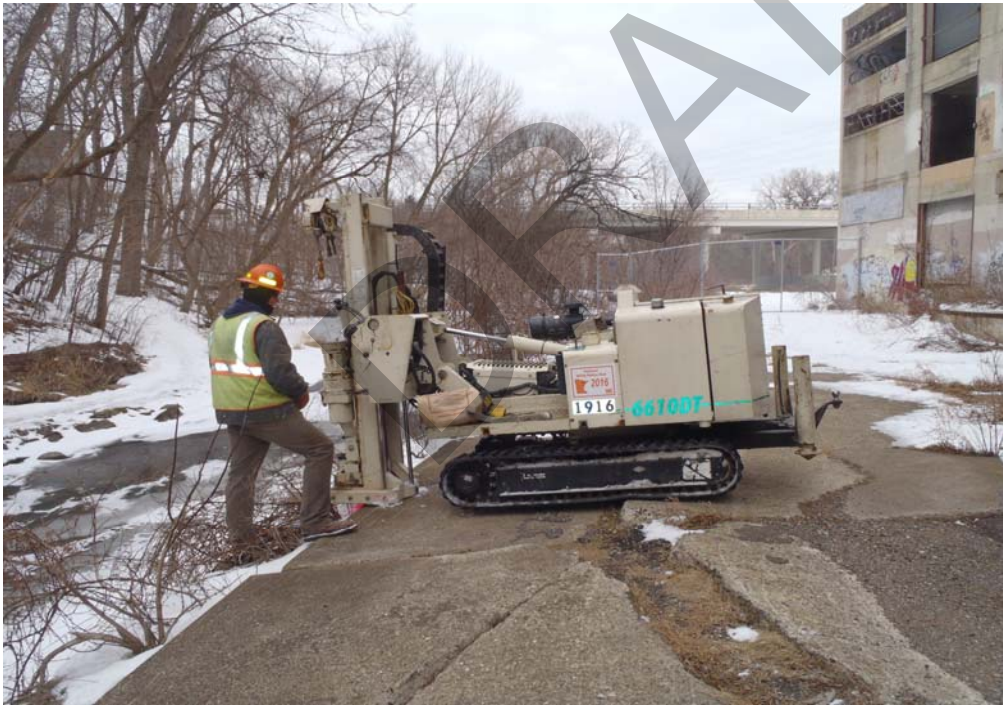
Photo 1: Geoprobe Setup at SB-15-01
