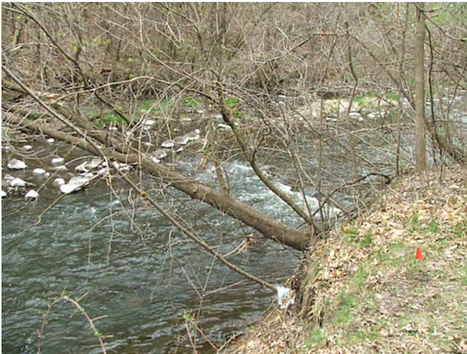
Photo 4: Eroded Retaining Wall “Rapids”.
