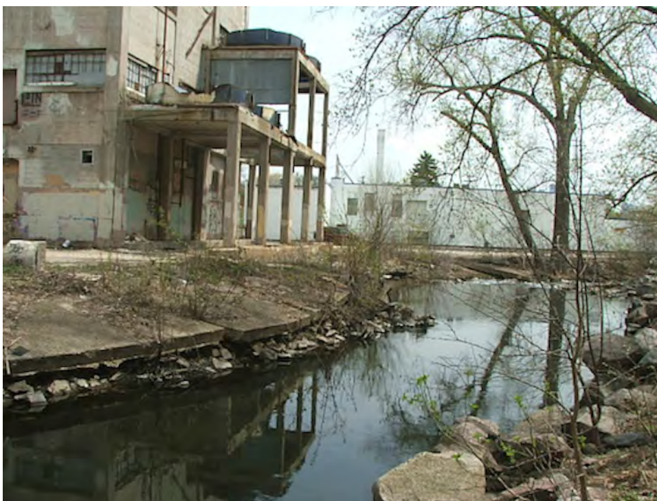
Photo 12: Downstream toward dam, Fruen Mill (right), and Glenwood-Inglewood Water Company (background).
