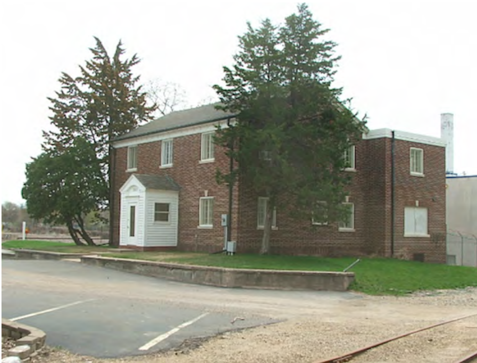
Photo 2: Glenwood-Inglewood Water Company Office Building.
