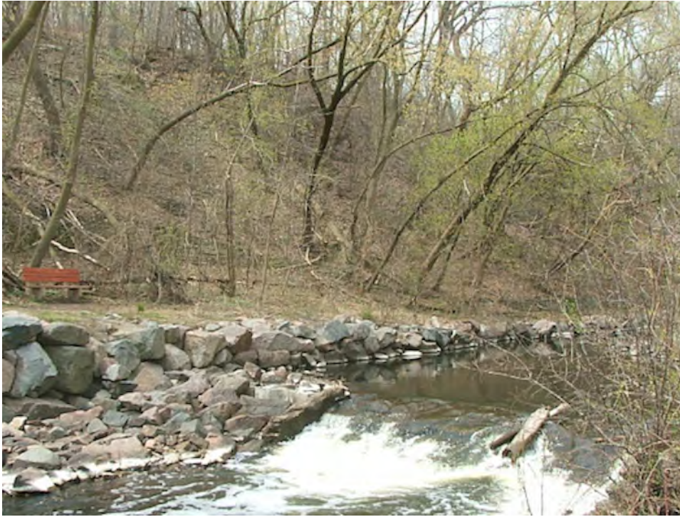
Photo 3: Rip Rap and Dam.
