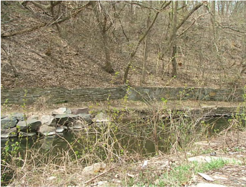
Photo 3: Bassett Creek Park Retaining Walls.
