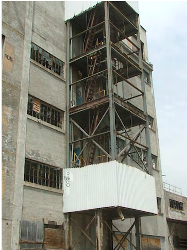
Photo 21: Fruen Mill Access Staircase.
