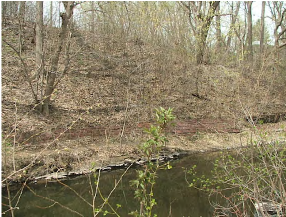
Photo 1: Bassett Creek Park Retaining Walls.
