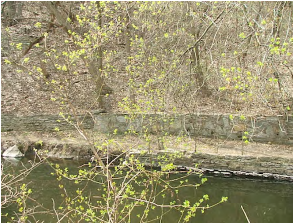
Photo 6: Bassett Creek Park Retaining Walls.
