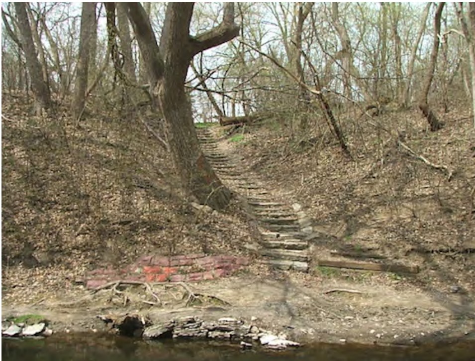
Photo 16: Bassett Creek Park Cut Stone Retaining Walls, Wooden Retaining Walls, and Stone Staircase.
