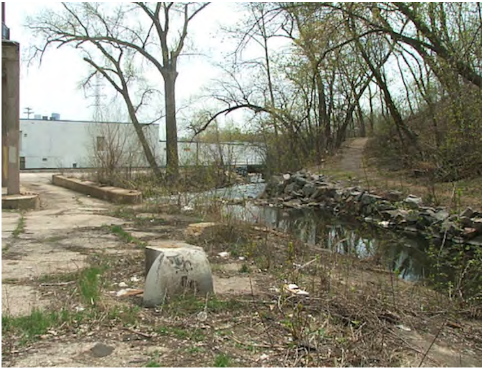
Photo 9: Looking Downstream From Mill Past Dam.
