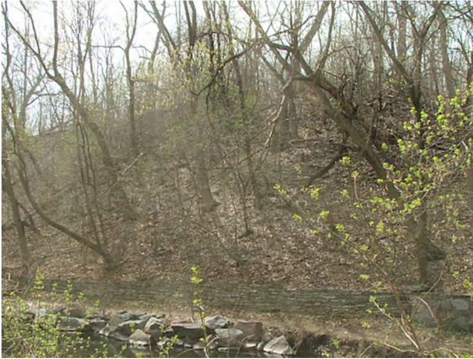
Photo 7: Bassett Creek Park Retaining Walls.
