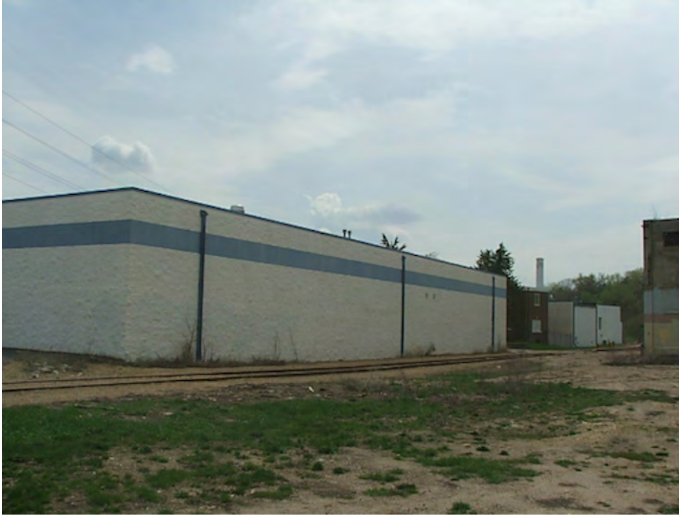
Photo 5: Glenwood-Inglewood Water Company and Railroad.
