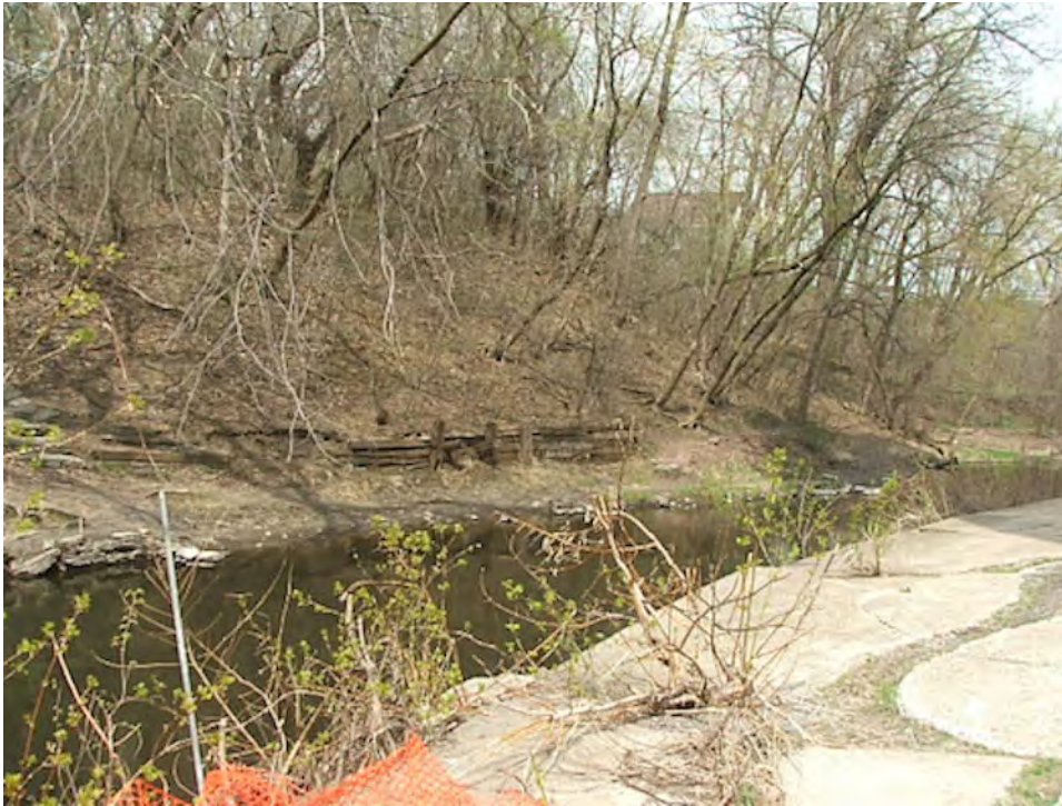
Photo 15: Bassett Creek Park Wooden Retaining Walls.
