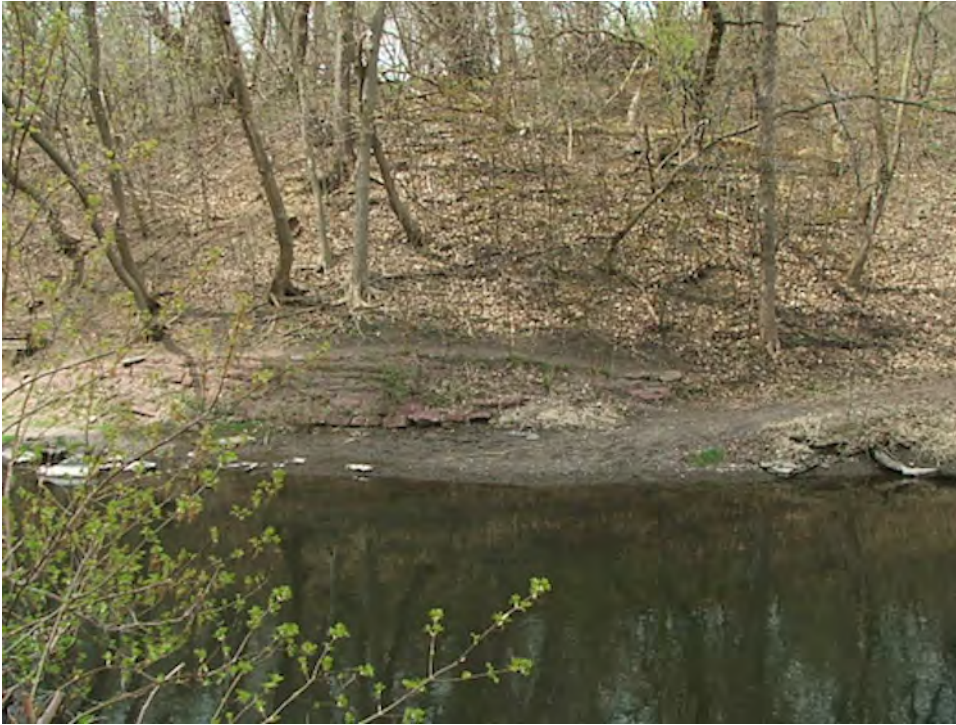
Photo 17: Bassett Creek Park Cut Stone Retaining Walls - note erosion.
