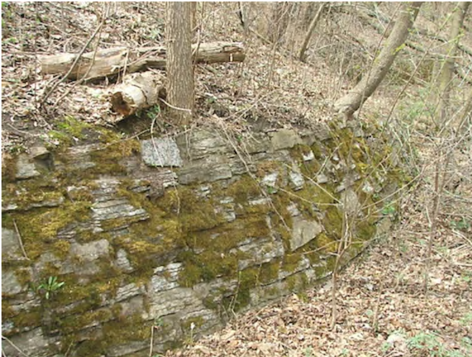
Photo 12: Bassett Creek Park Retaining Wall (detail).
