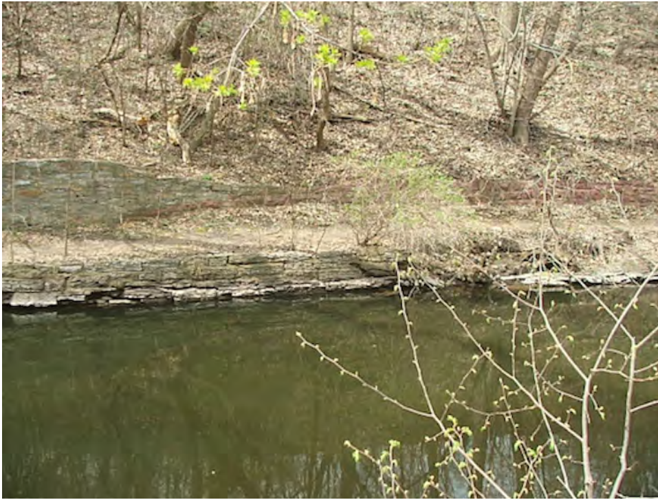
Photo 5: Bassett Creek Park Retaining Walls.
