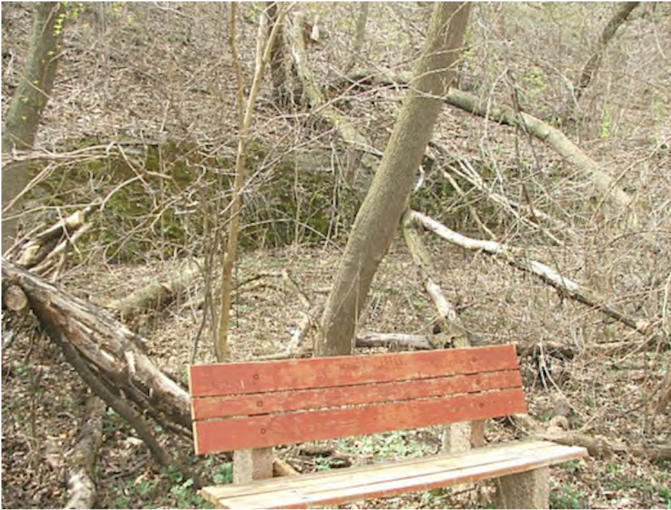
Photo 13: Bassett Creek Park Bench and Retaining Walls.
