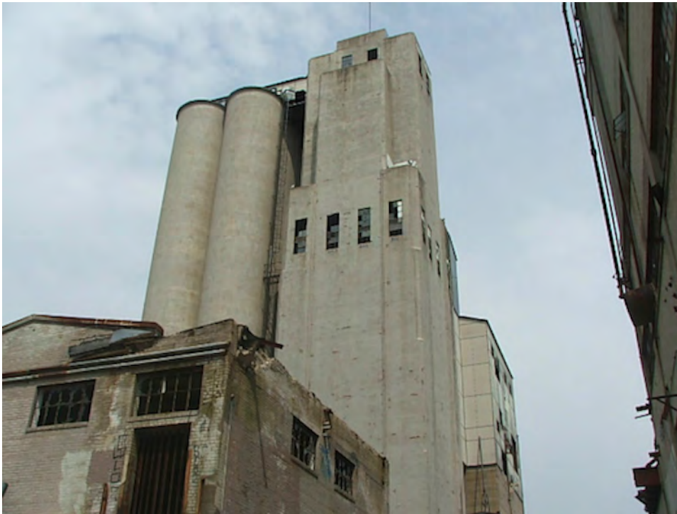
Photo 6: Fruen Mill Grain Silos and Elevator.
