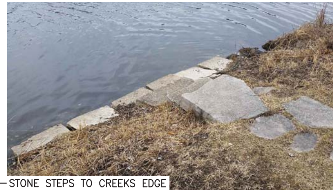
STONE STEPS TO CREEK'S EDGE
