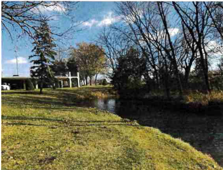
View of creek channel bank and current water level (photo facing south).
