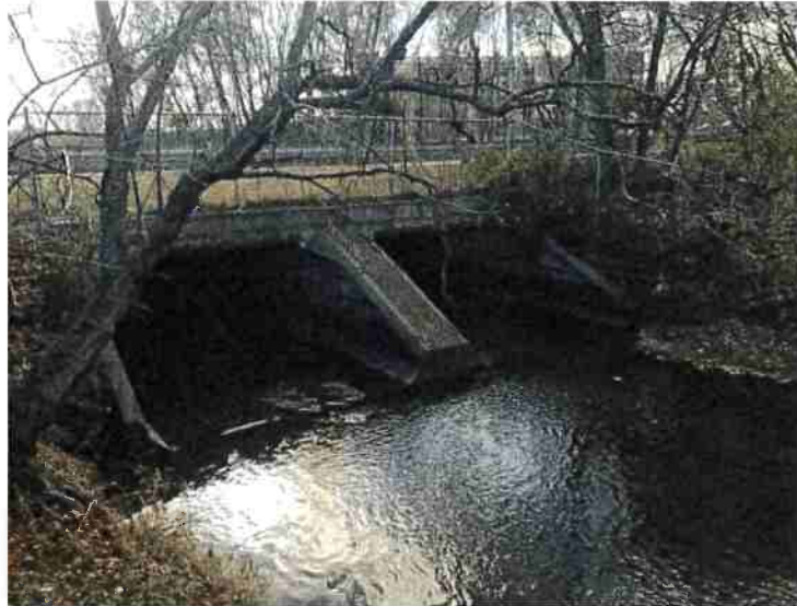
Box culvert under frontage road (photo facing south).
