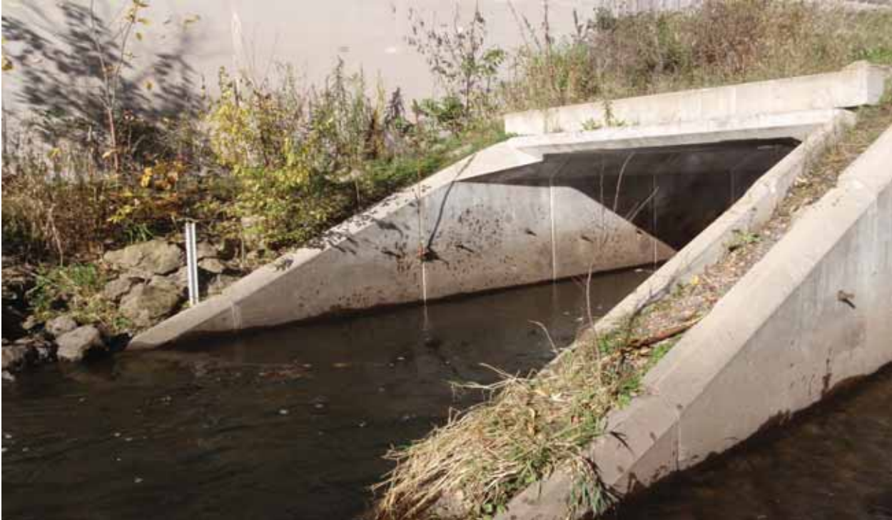
Highway 100 Double Box Culvert (Crystal/Golden Valley)
