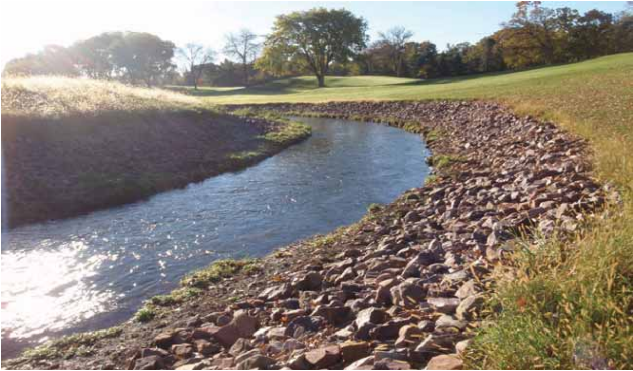
Golden Valley Country Club Control Structure (US Channel)
