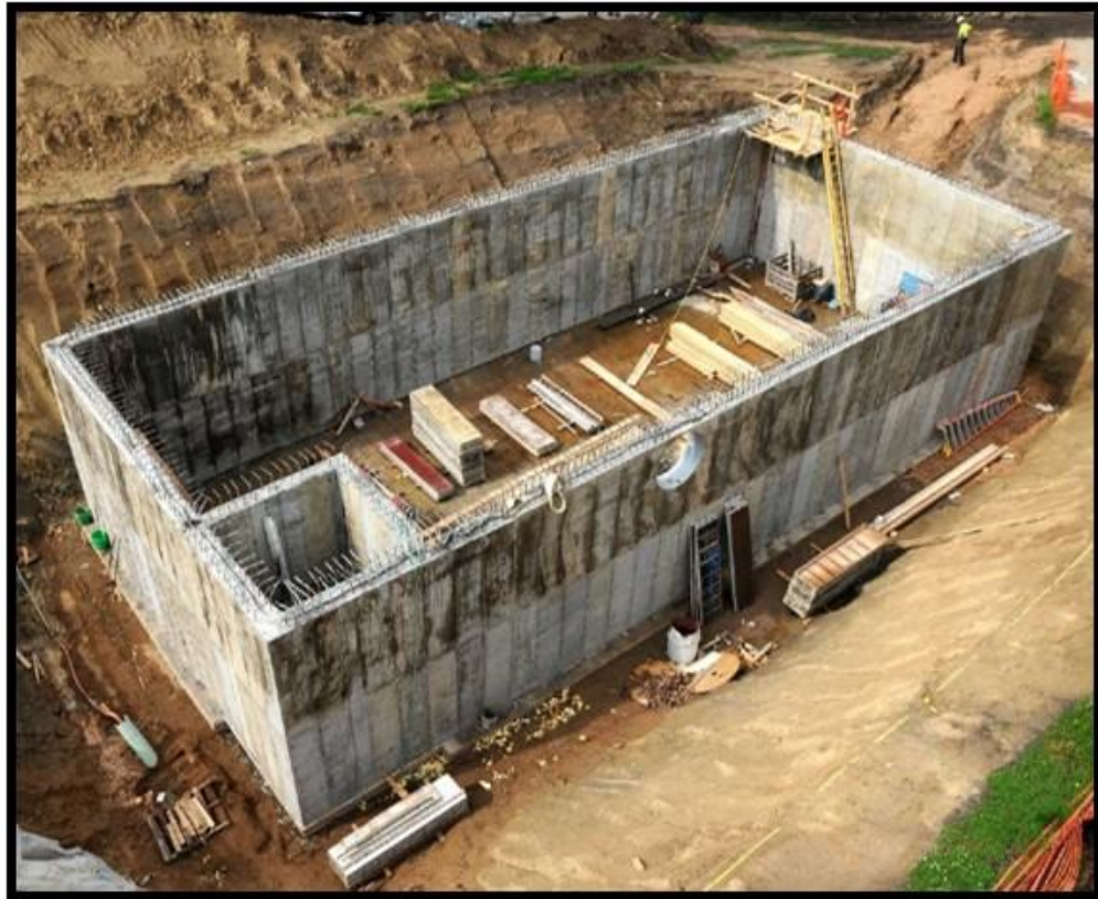
Underground Storm Water Reuse Tank
