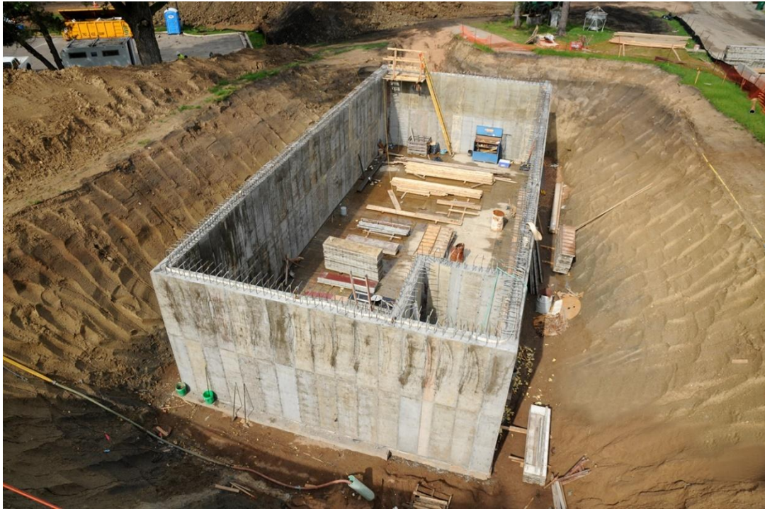
Underground Storm Water Reuse Tank
