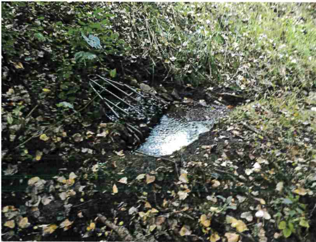
View of culvert leading in to Wetland 1 near W1-2W.
