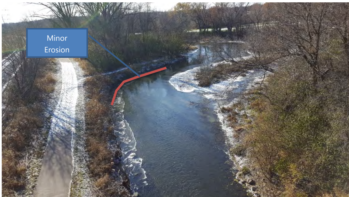
Figure 3-6 Project reach downstream of Plymouth Ave. N bridge (minor erosion in the left overbank)
