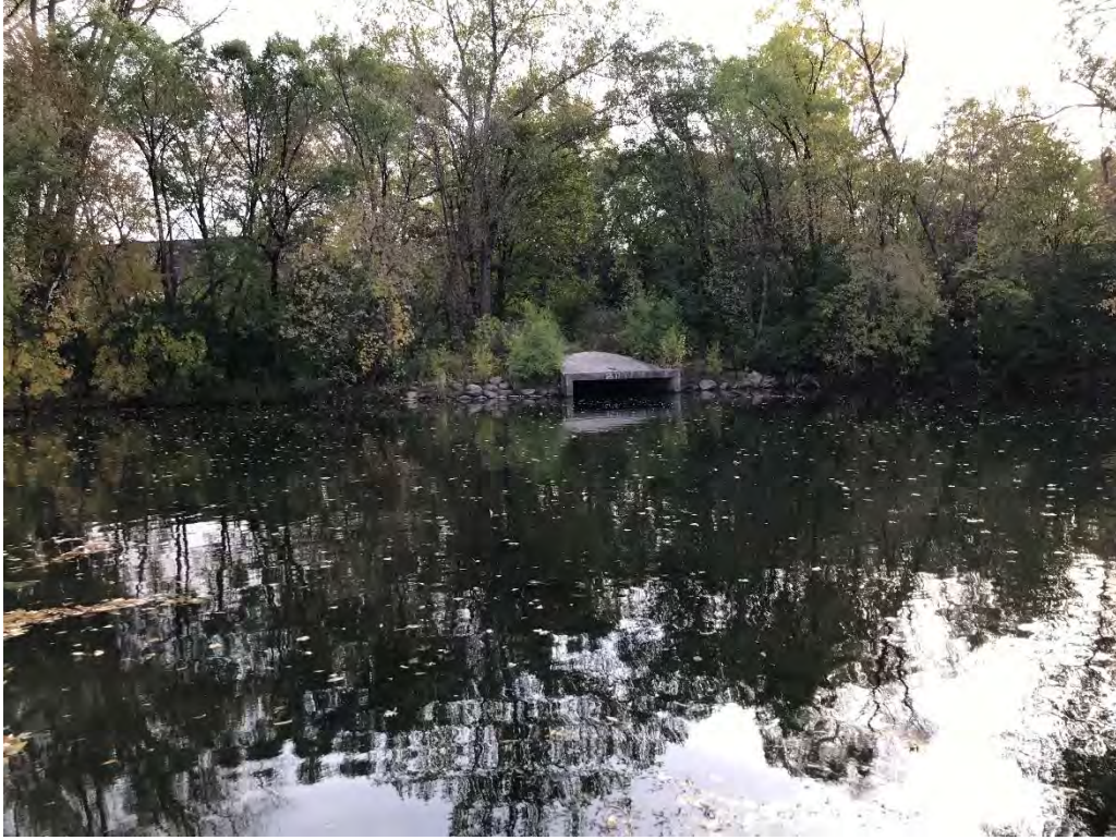
Photograph #9: Lagoon E – Culvert near LE-SED-01
