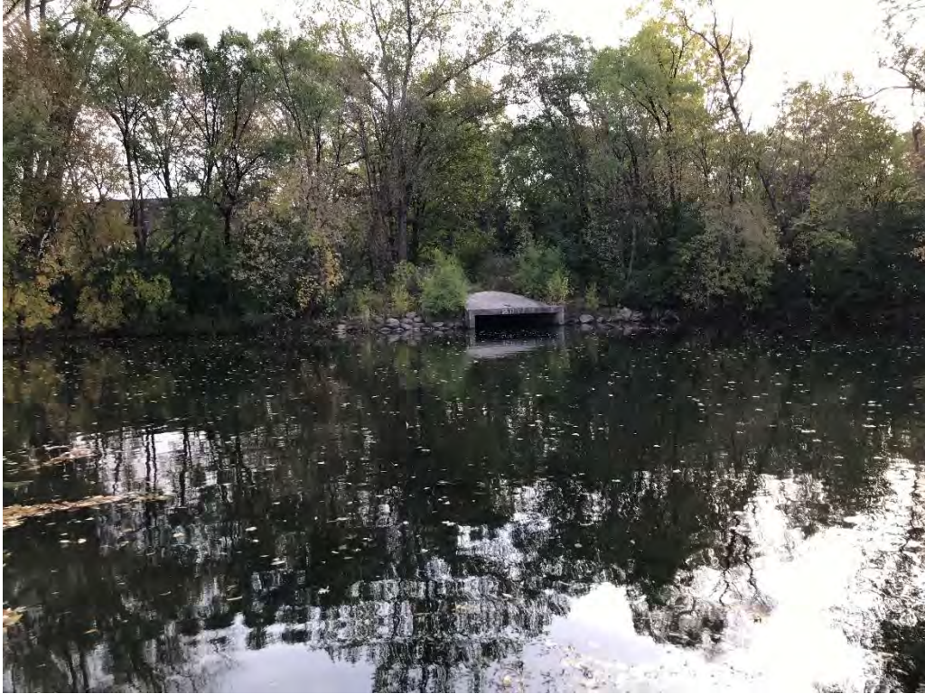
Photograph #9: Lagoon E – Culvert near LE-SED-01
