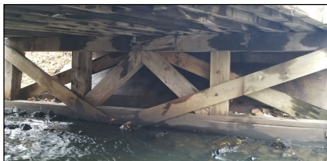
North Bridge Abutment
