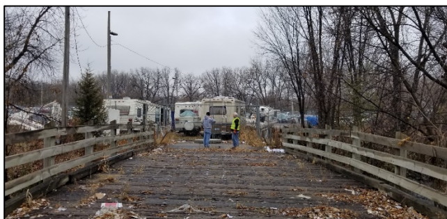
Irving Ave Bridge Deck
