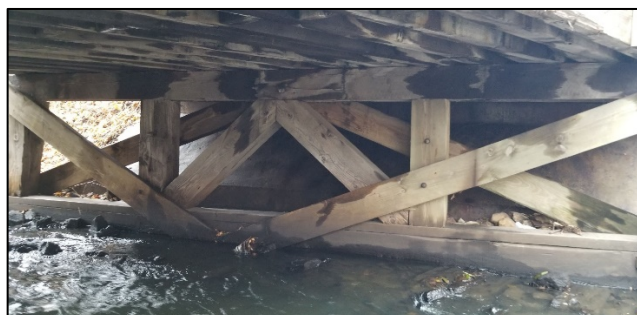
North Bridge Abutment
