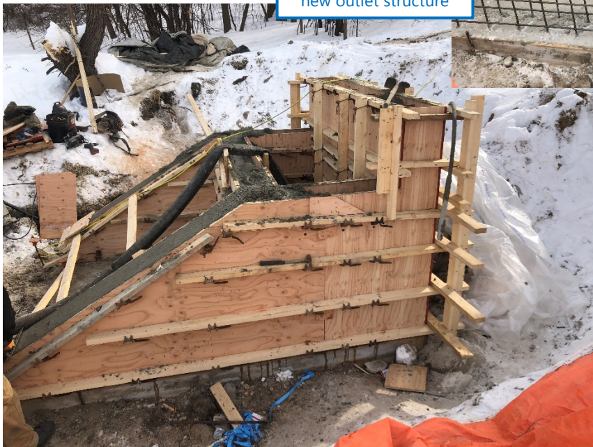
Forming and pouring new outlet structure
