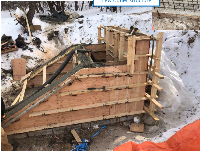
Forming and pouring new outlet structure
