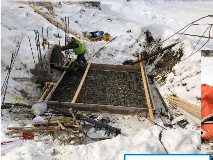
Forming and pouring new outlet structure
