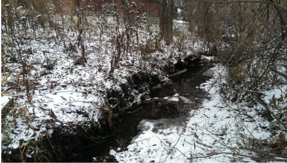
Figure 3-8 Parkers Lake Erosion Example
