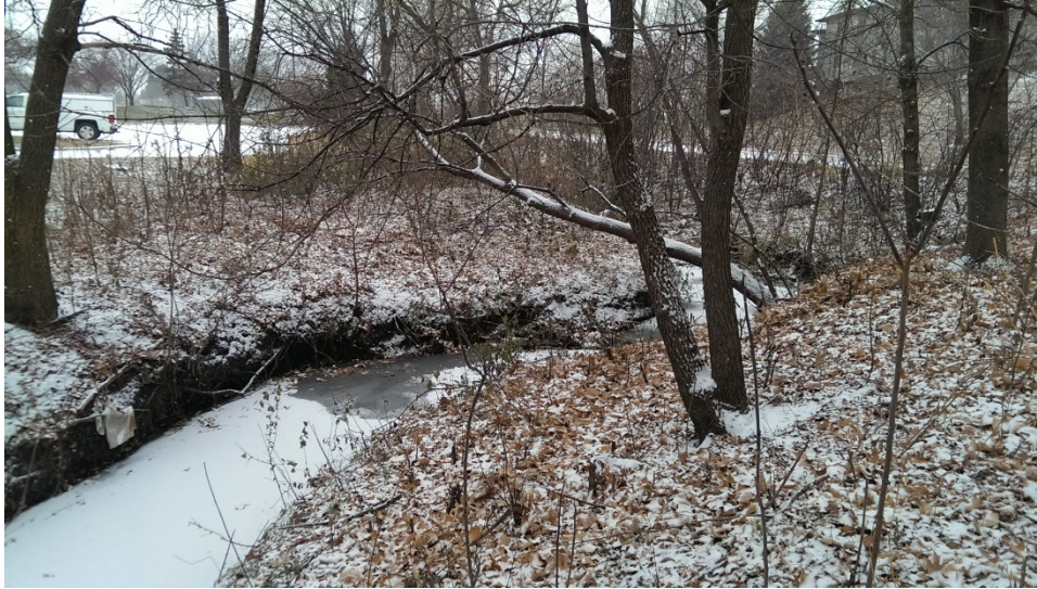
Figure 3-6 Parkers Lake Erosion Example
