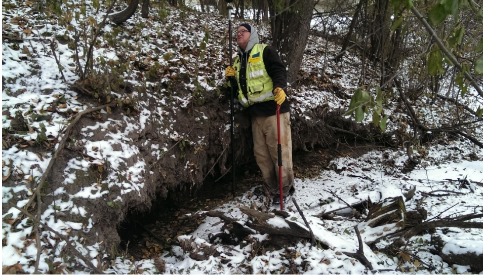
Figure 3-4 Mount Olivet Erosion Example (bank erosion)
