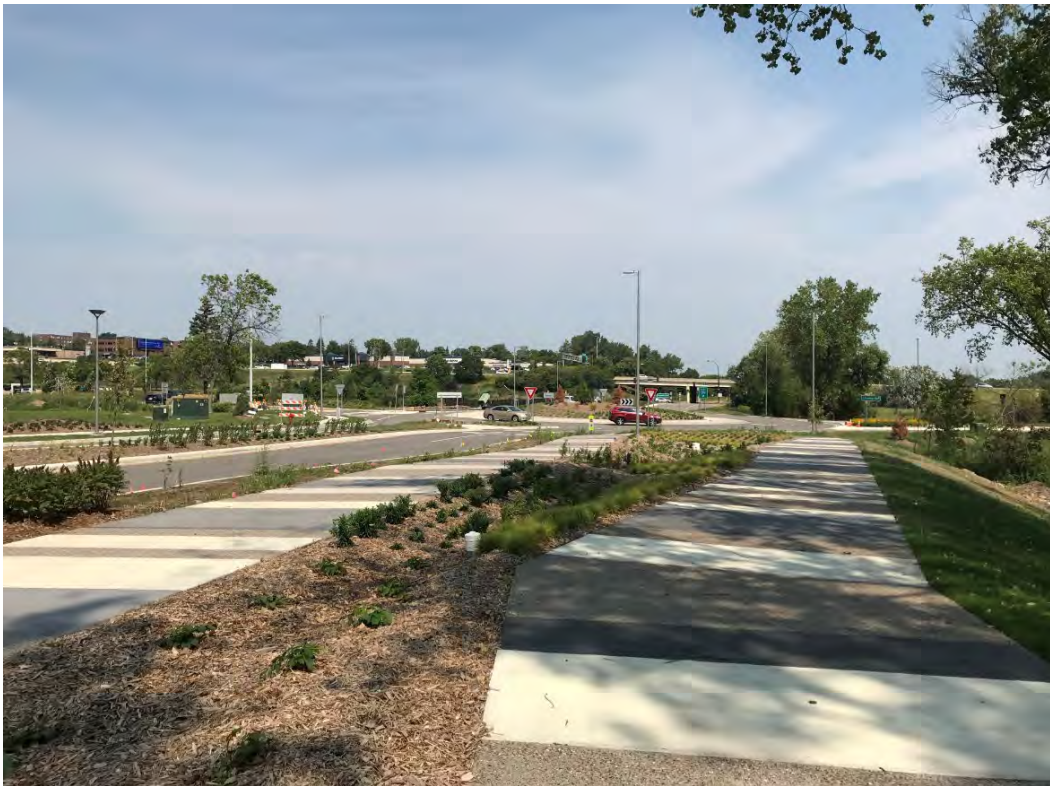
South Rain Garden Plantings Installed – North View
