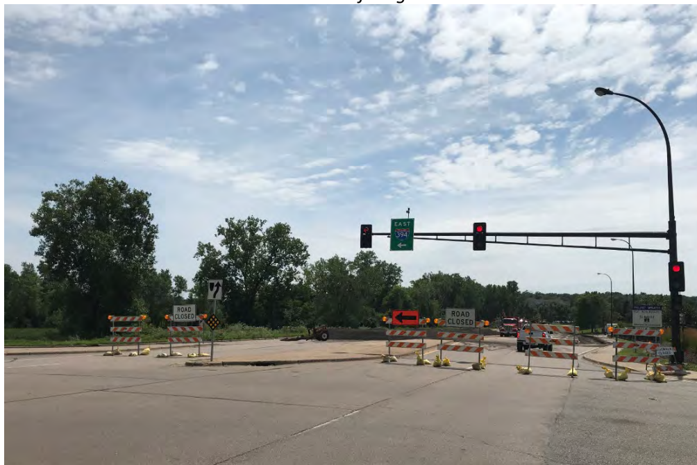
Construction Starting - South View of Ridgedale Drive & Crane Lake Park
