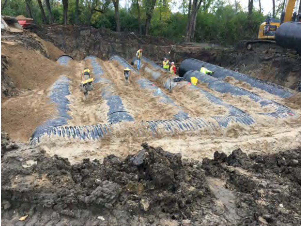
Underground Storm Water Tank Construction at Crane Lake Park – East View
