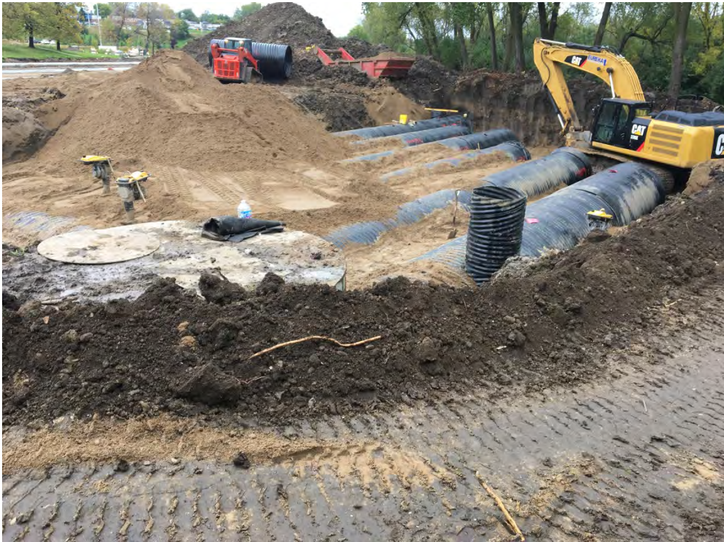
Underground Storm Water Tank Construction at Crane Lake Park – North View
