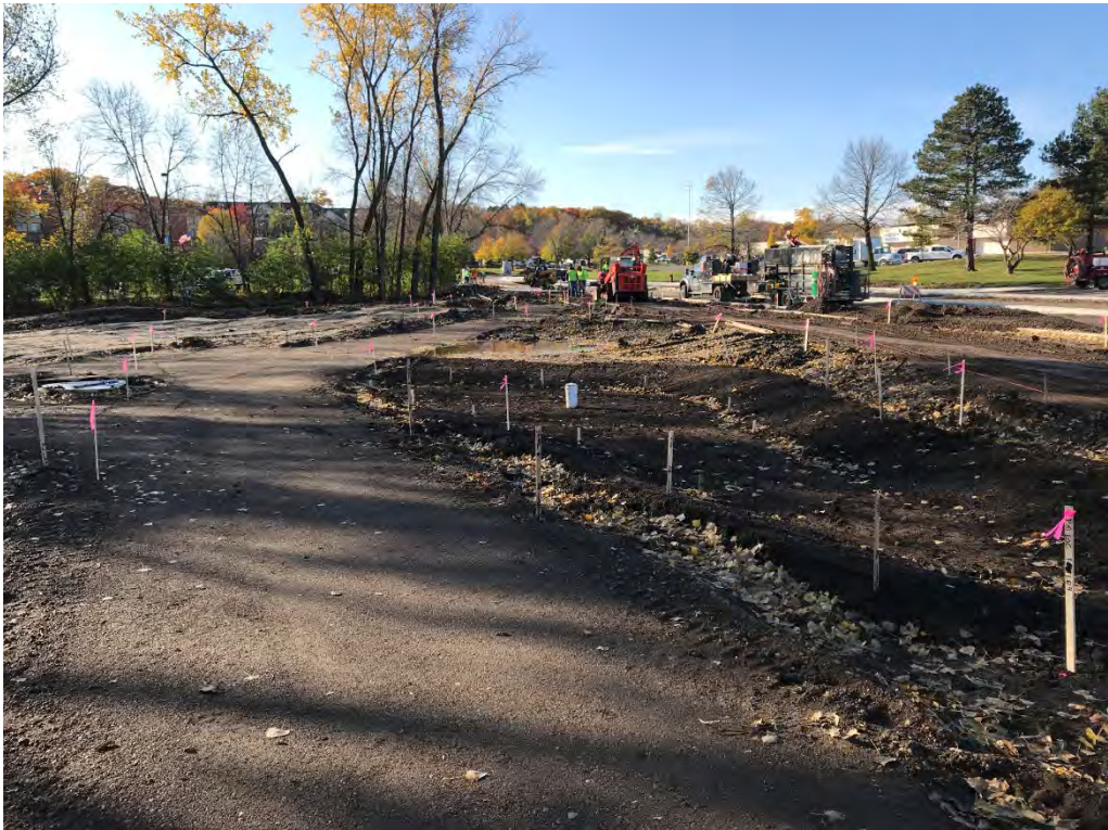
South Rain Garden – South View
