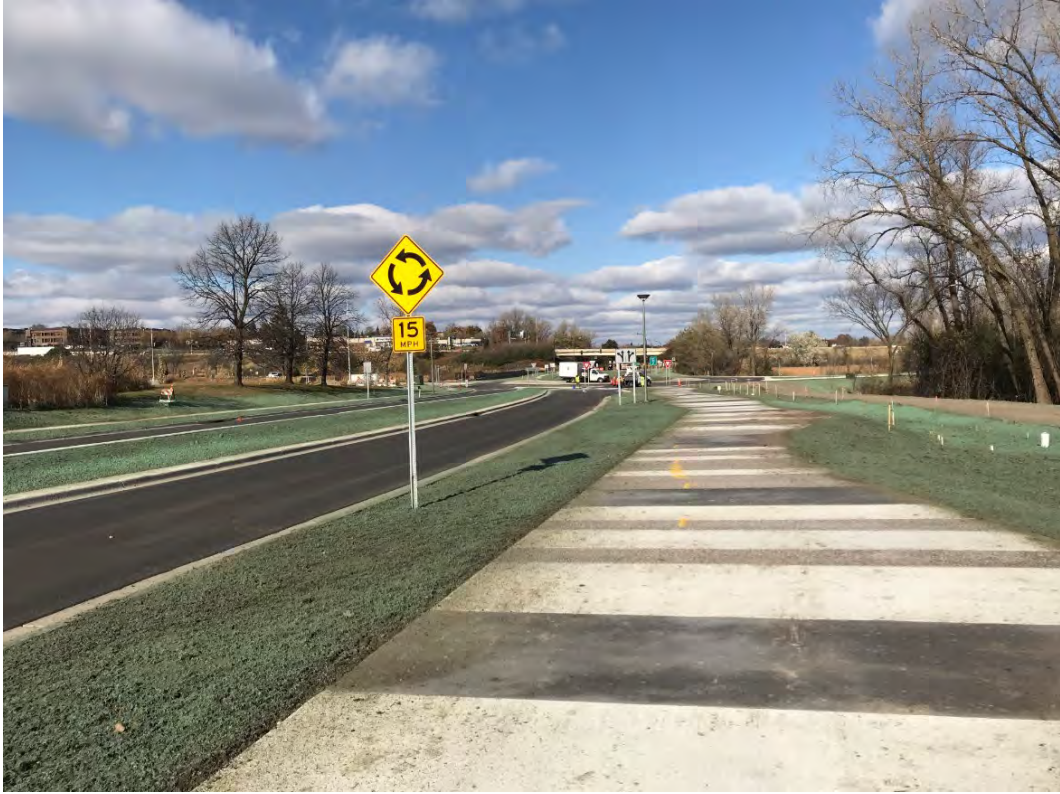
Temporary Seeding – North View
