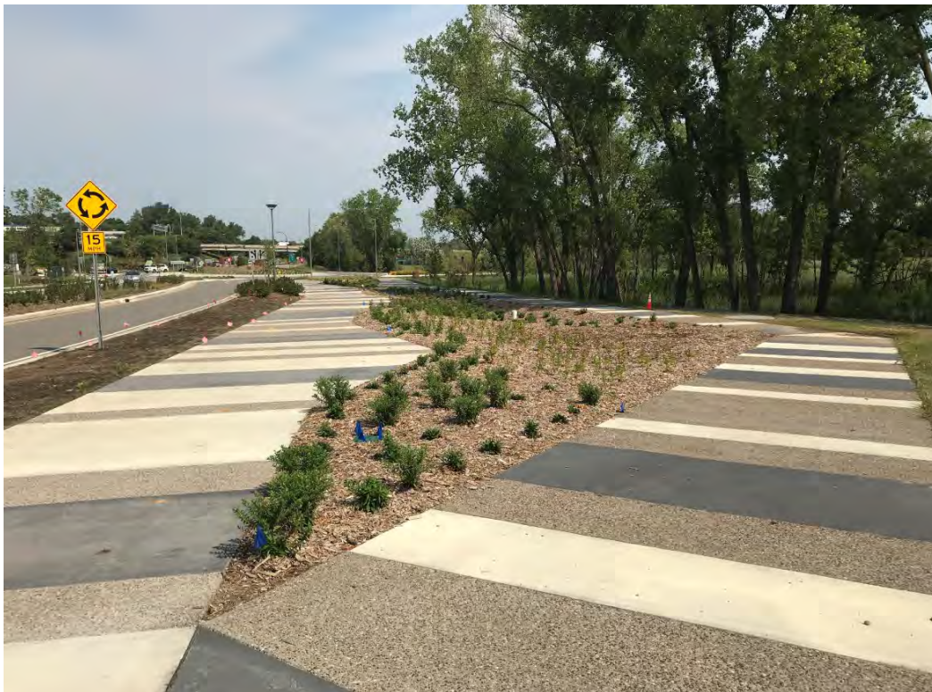
North Rain Garden Plantings Installed – North View
