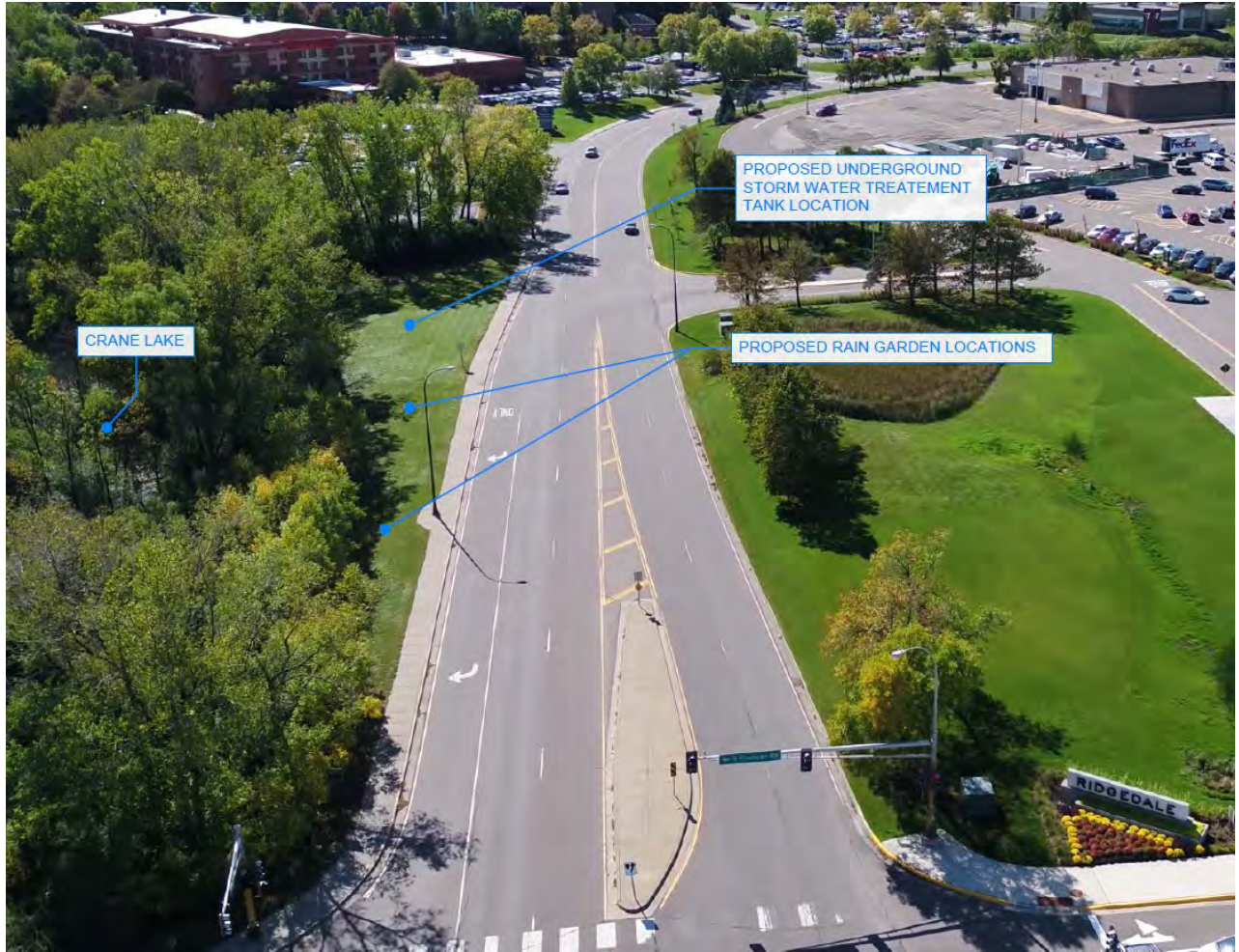
Preconstruction - Drone South View of Ridgedale Drive & Crane Lake Park
