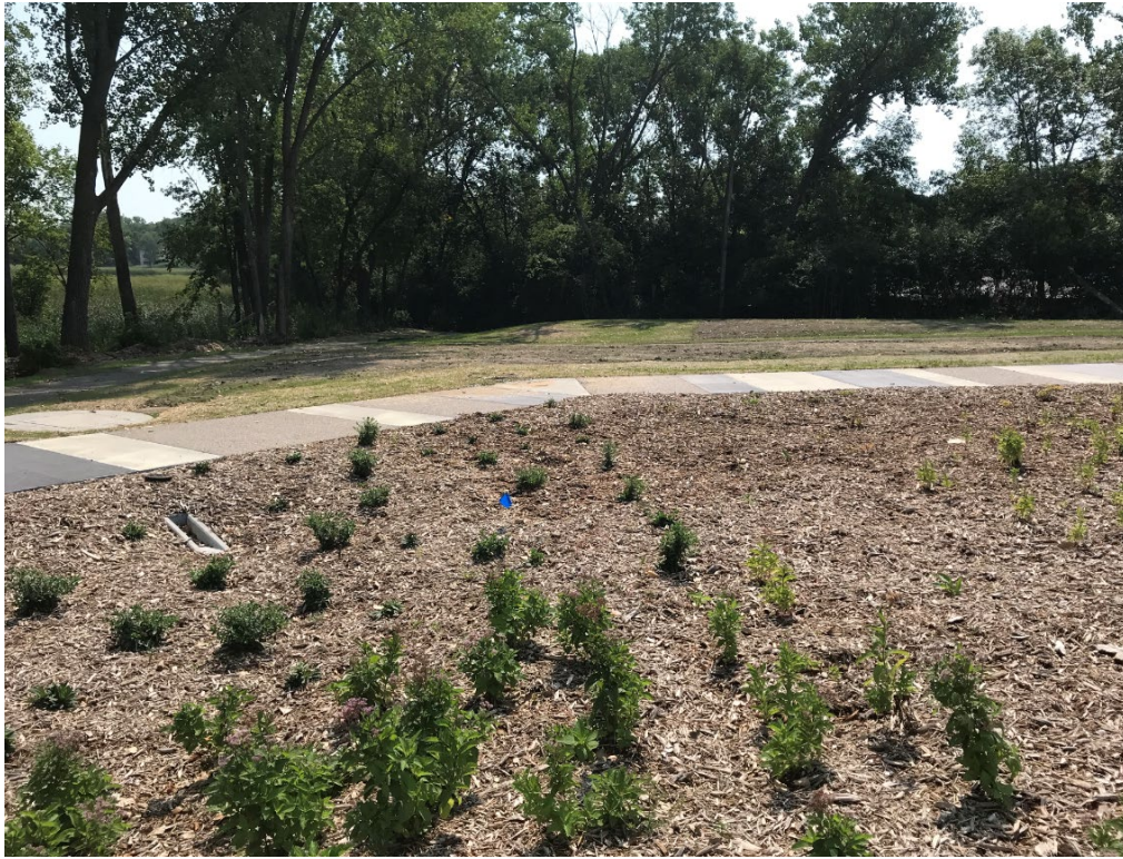
North Rain Garden Plantings Installed (Lift Station Outlet Left Side of Photo) – SE View
