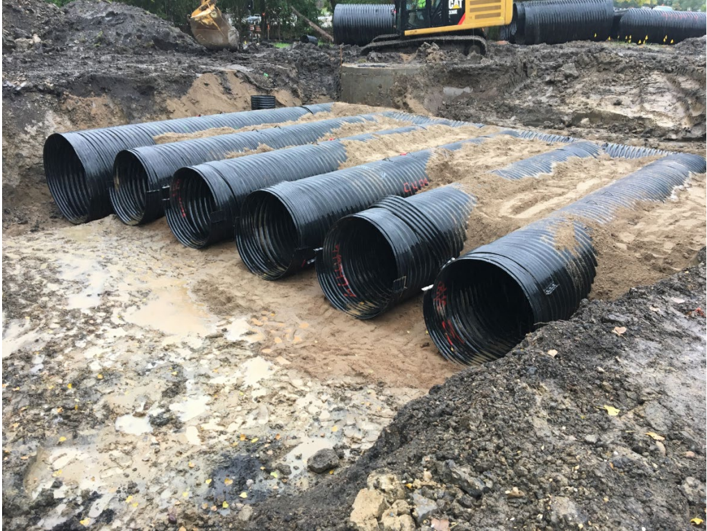
Underground Storm Water Tank Construction at Crane Lake Park – South View
