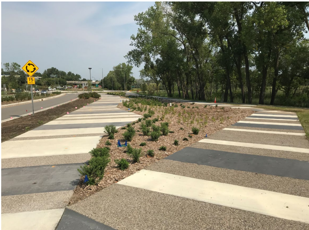
North Rain Garden Plantings Installed – North View
