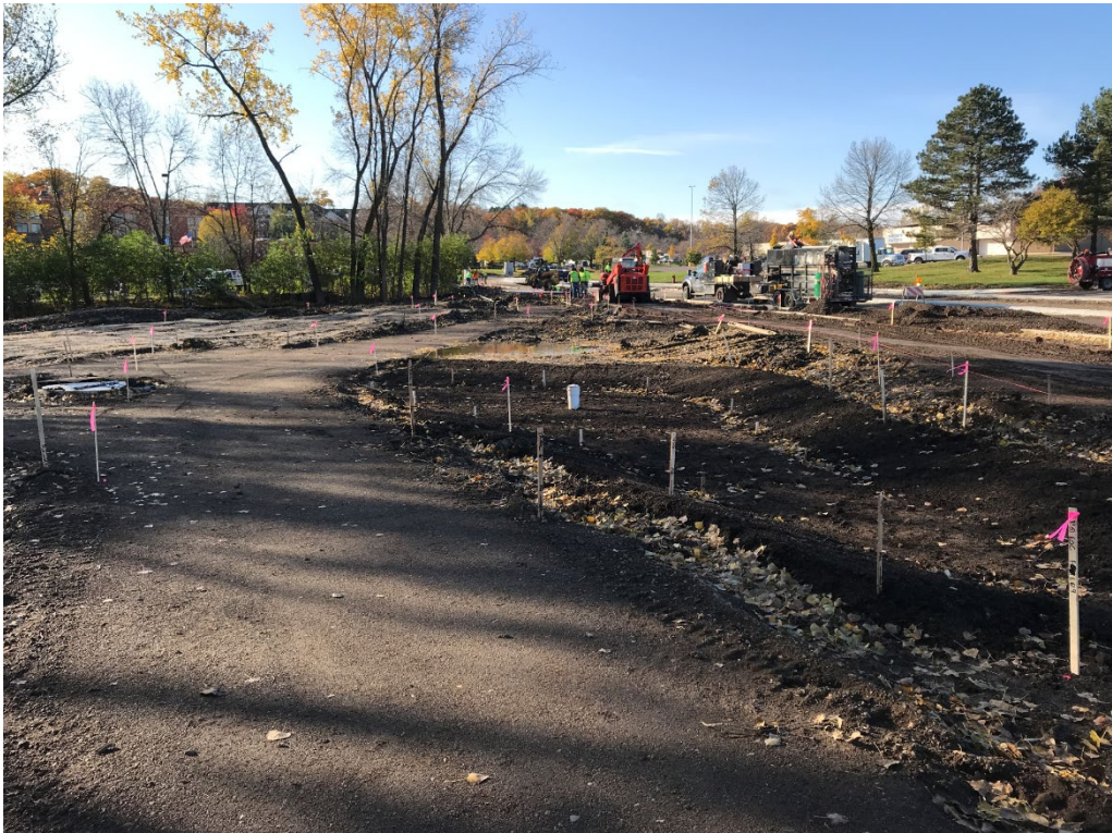
South Rain Garden – South View
