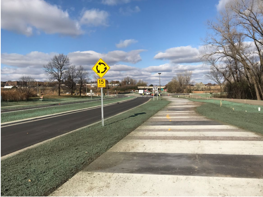
Temporary Seeding – North View
