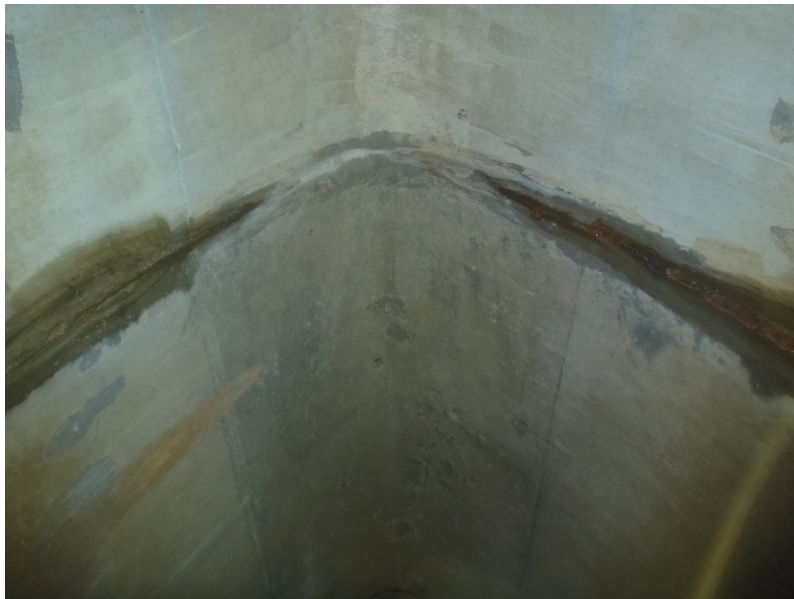
infiltration weeper
