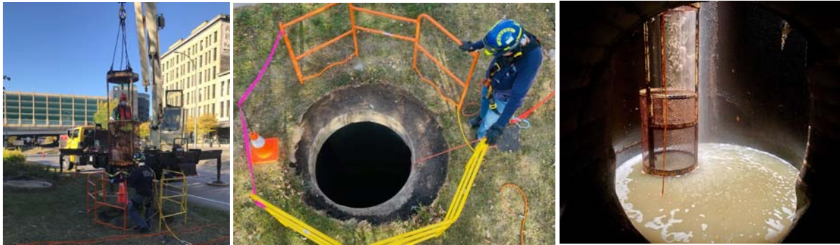
Figure 3-2 Washington Avenue Shaft
