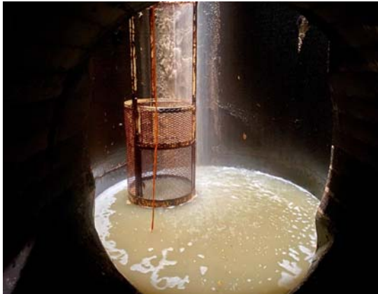
Figure 6-2 Washington Avenue Shaft
