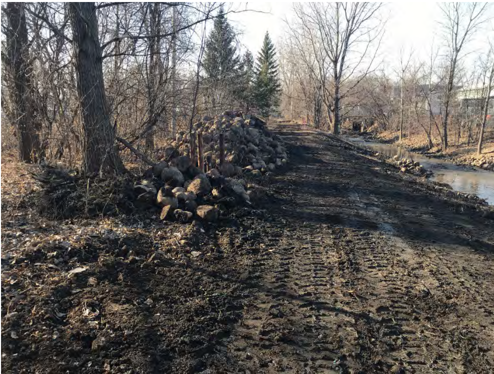
Reach 1: Cleared southern bank downstream of Irving Ave. footbridge (12/10/2020)
