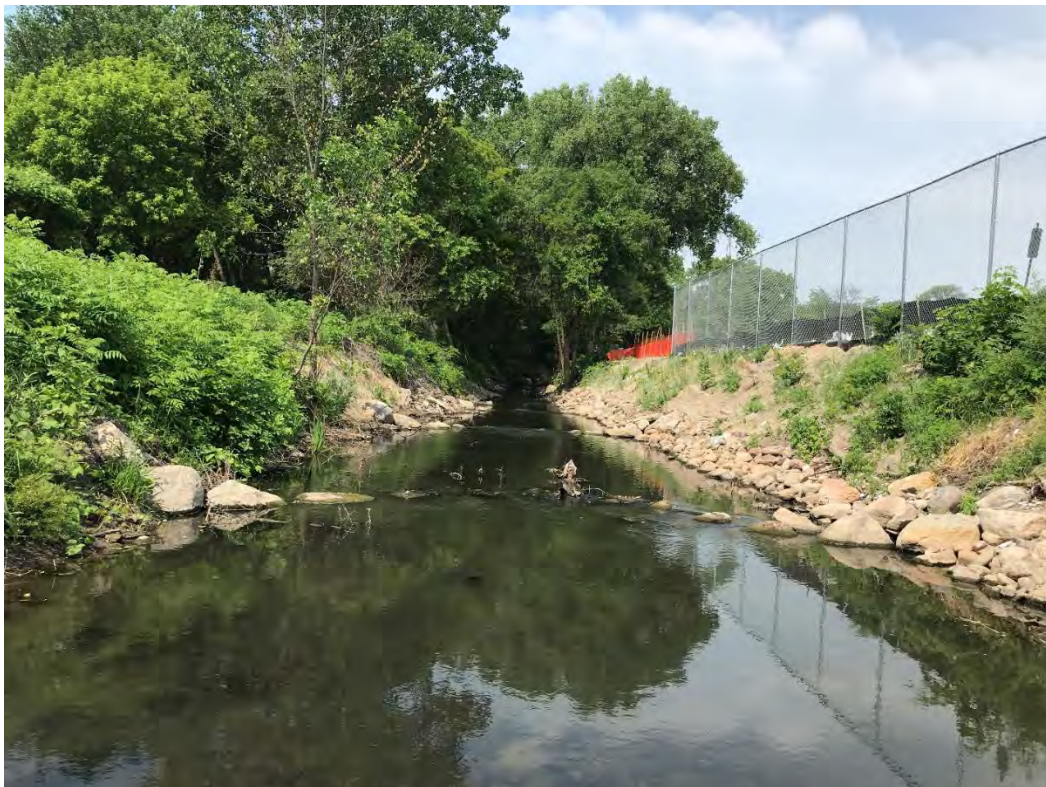
Reach 1: Upstream boulder vanes and riprap (6/17/2021)
