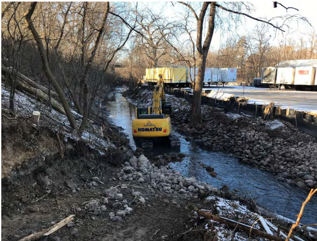
Reach 1: Installation of upstream riprap and boulder vanes (12/14/2020)
