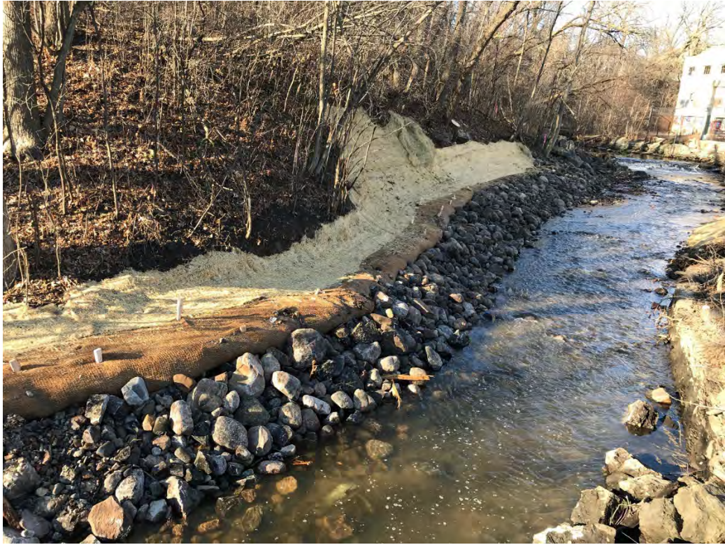
Reach 2: Installed riprap, erosion control blanket, and VRSS (12/4/2020)
