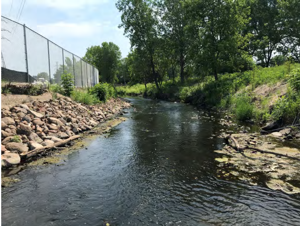
Reach 1: Riprap and native vegetation reestablishment upstream of Irving Ave. footbridge (6/17/2021)
