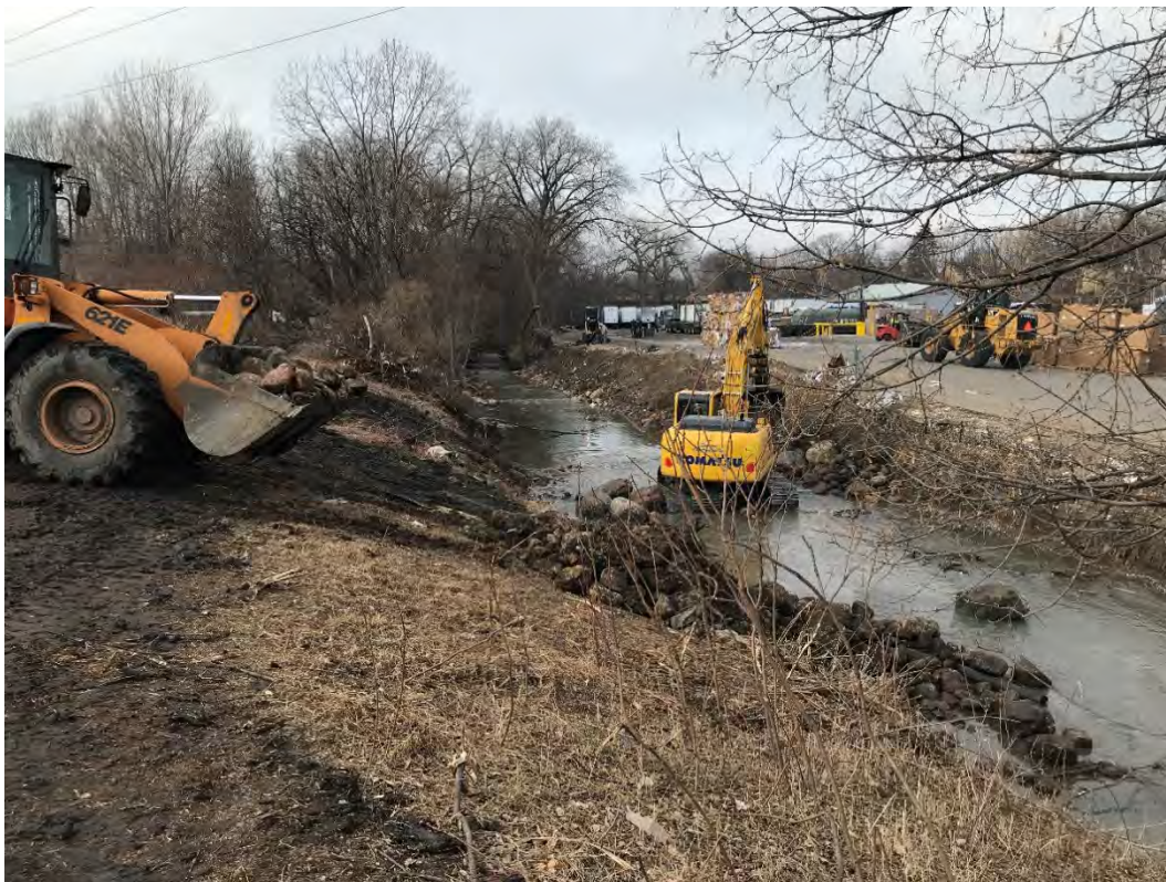
Reach 1: Installation of downstream boulder vanes (12/8/2020)
