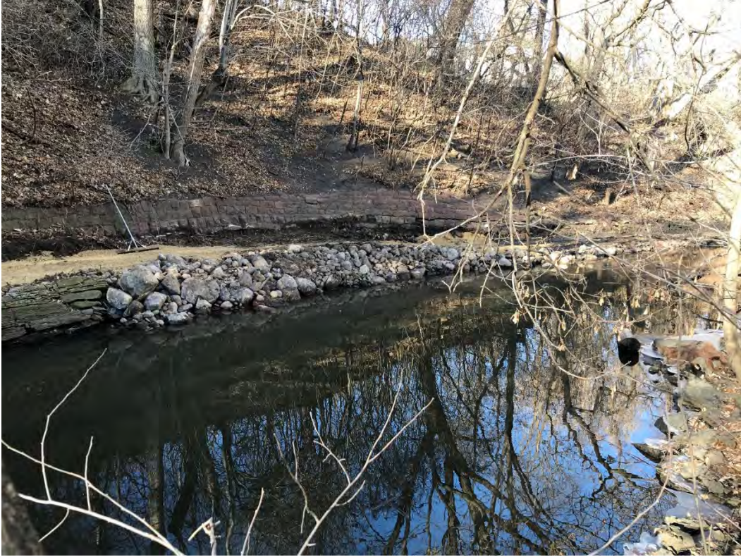
Reach 2: Installed riprap and trail improvement (12/4/2020)
