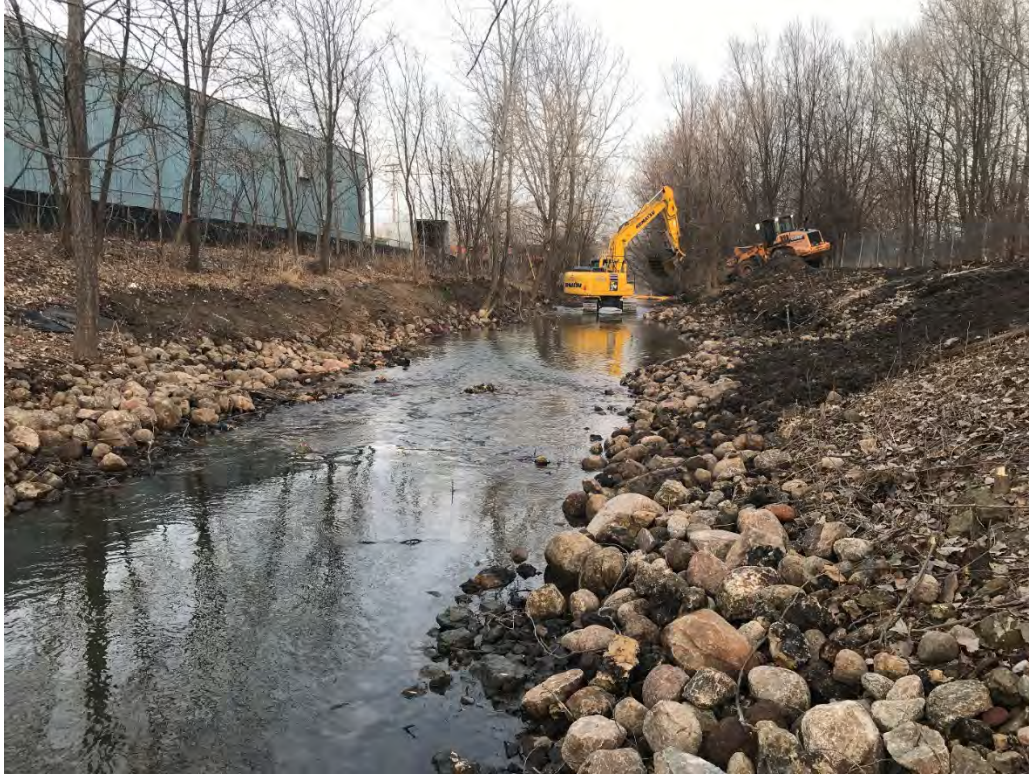
Reach 1: Installation of riprap downstream of Irving Ave. footbridge (12/10/2020)
