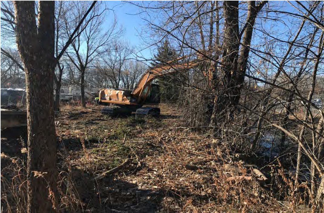
Reach 1: Tree and shrub clearing along the southern bank upstream of the Irving Ave. footbridge (12/1/2020)
