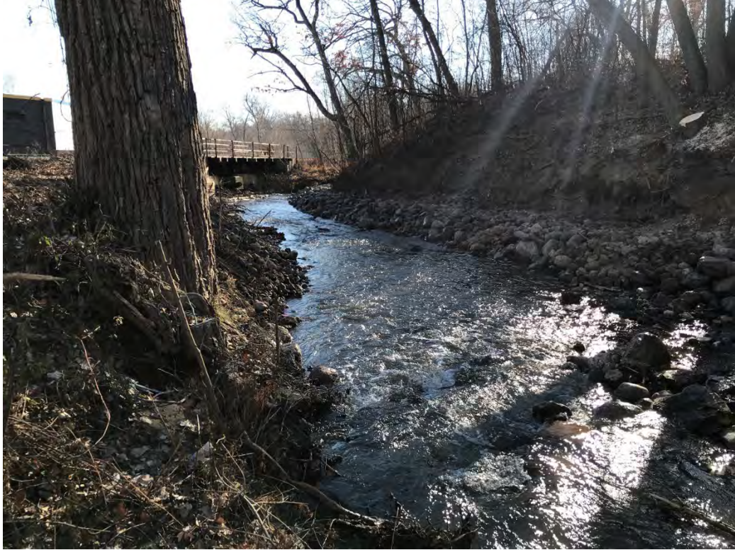
Reach 2: Installed riprap on downstream portion of the reach (12/1/2020)
