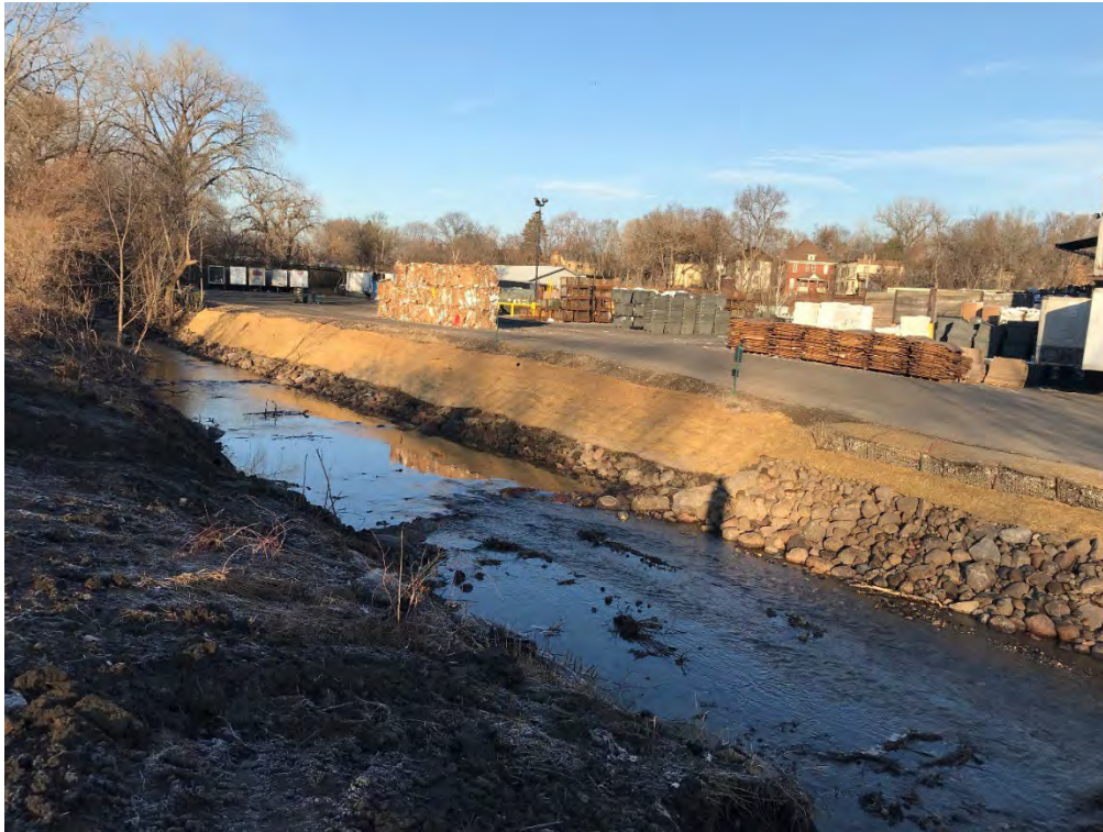
Reach 1: Installed riprap and erosion control blanket along northern bank (12/10/2020)
