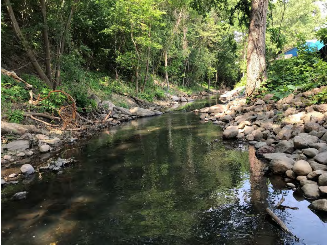
Reach 1: Upstream boulder vanes and riprap (6/17/2021)
