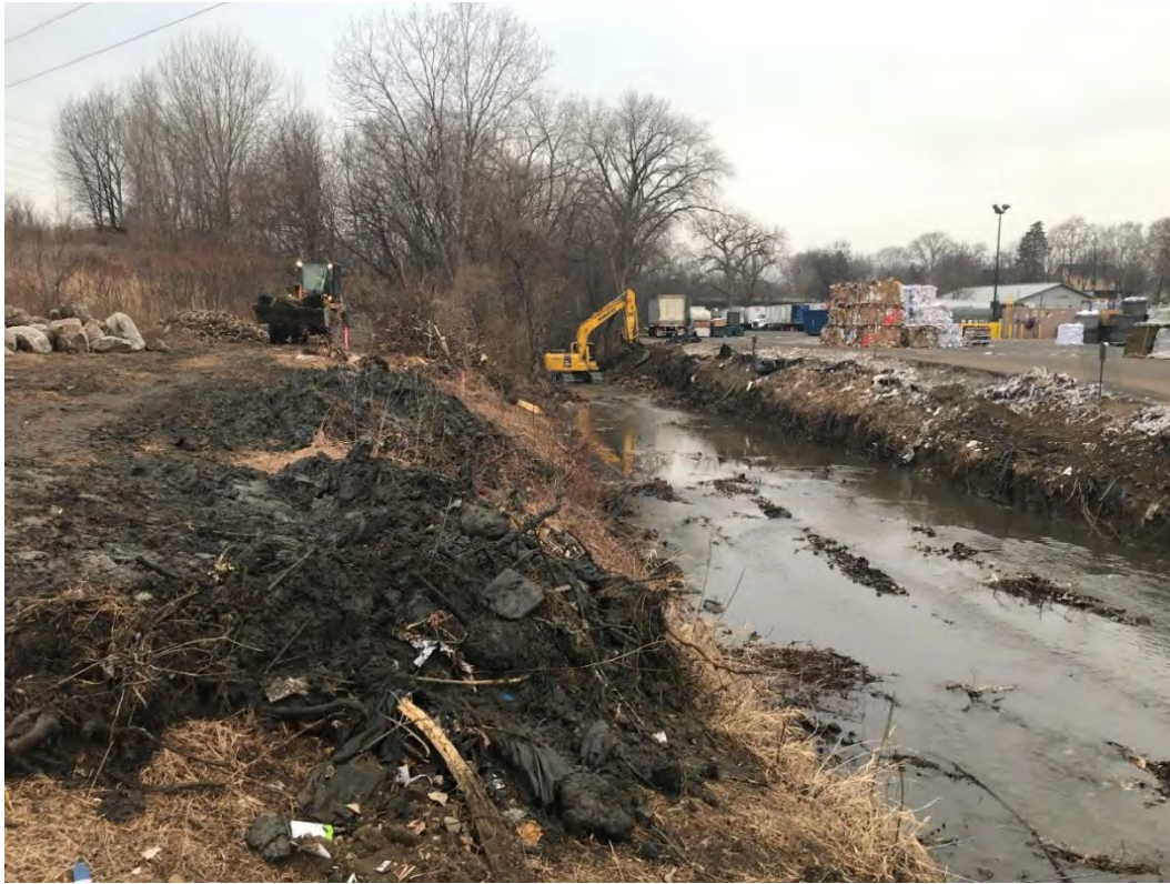
Reach 1: Removal of debris within the channel and installation of riprap (12/7/2020)
