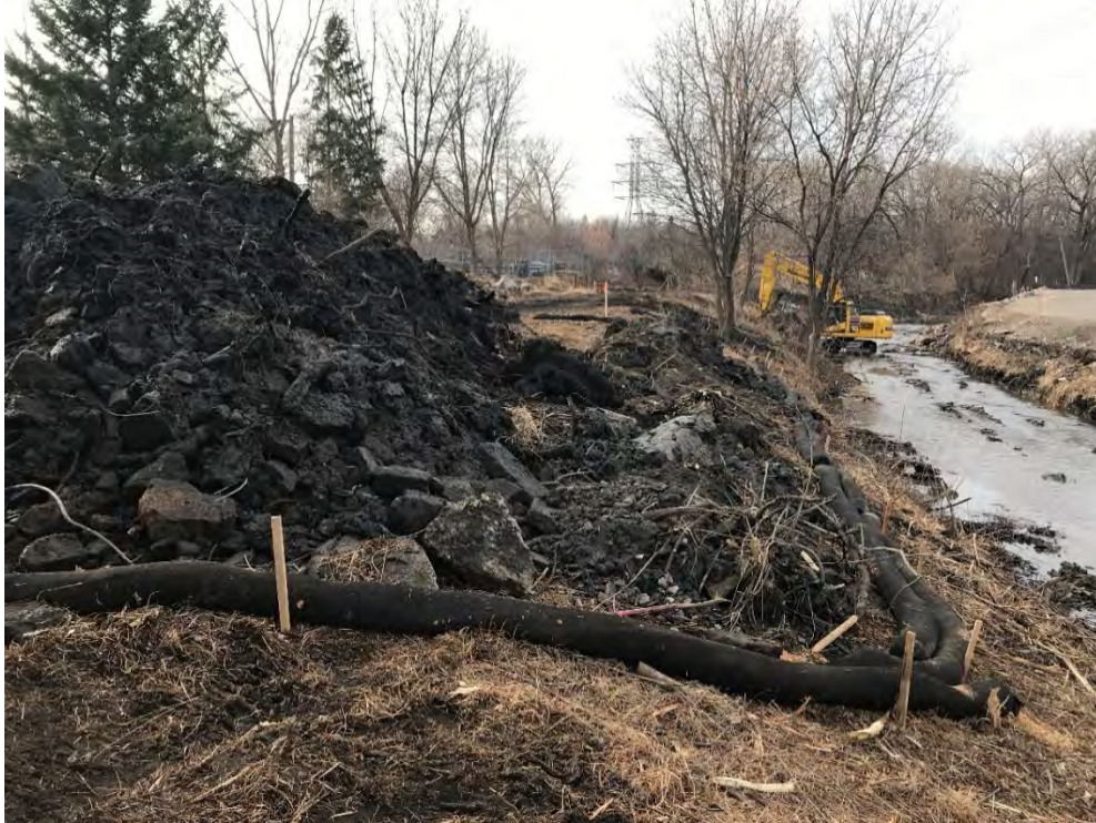
Reach 1: Stockpile of debris and contaminated soils with erosion control logs (12/8/2020)
