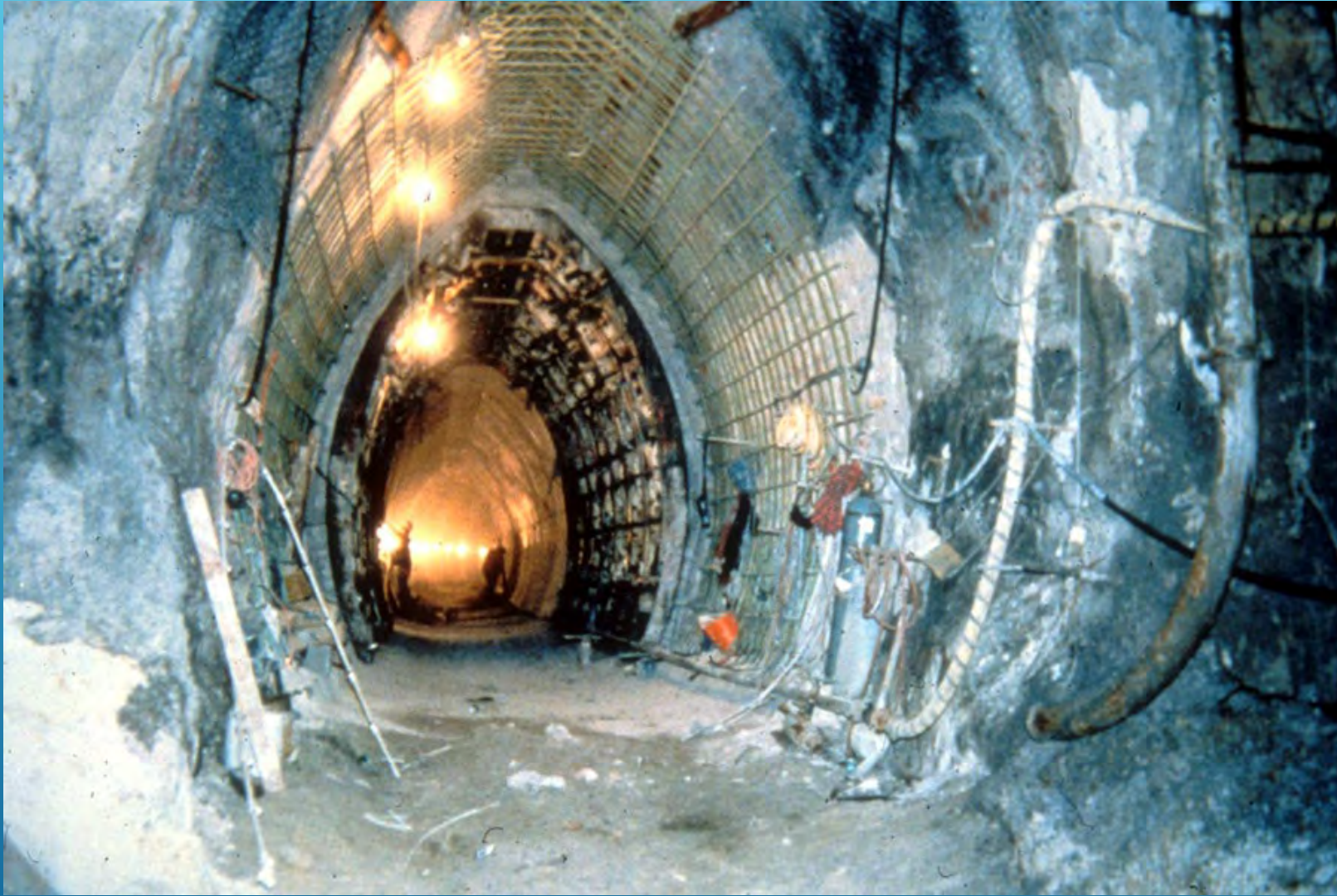
Bassett Creek Tunnel Construction 1978
