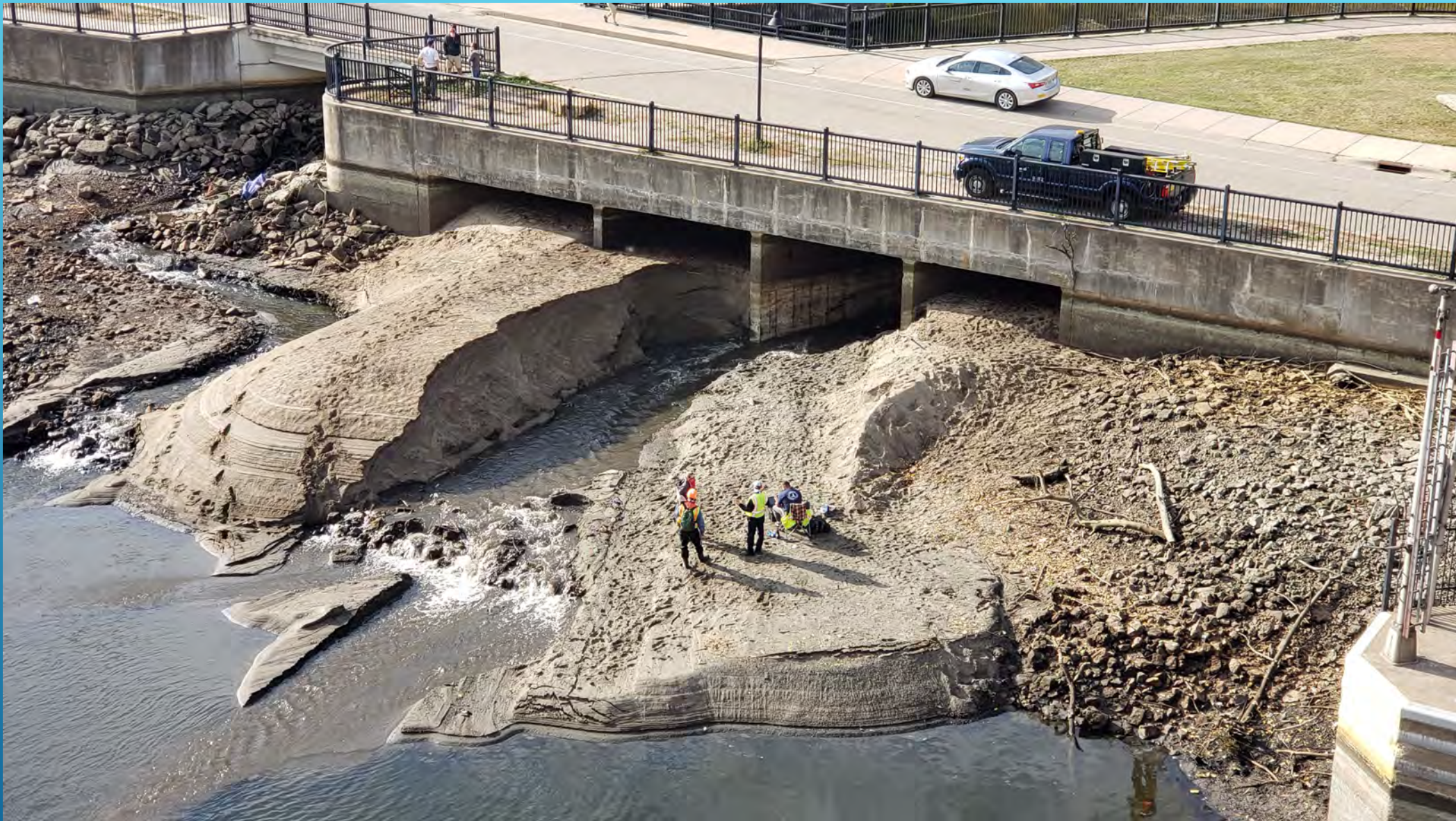
Bassett Creek Tunnel Outlet @ Mississippi River Drawdown and tunnel inspection – Fall 2020
