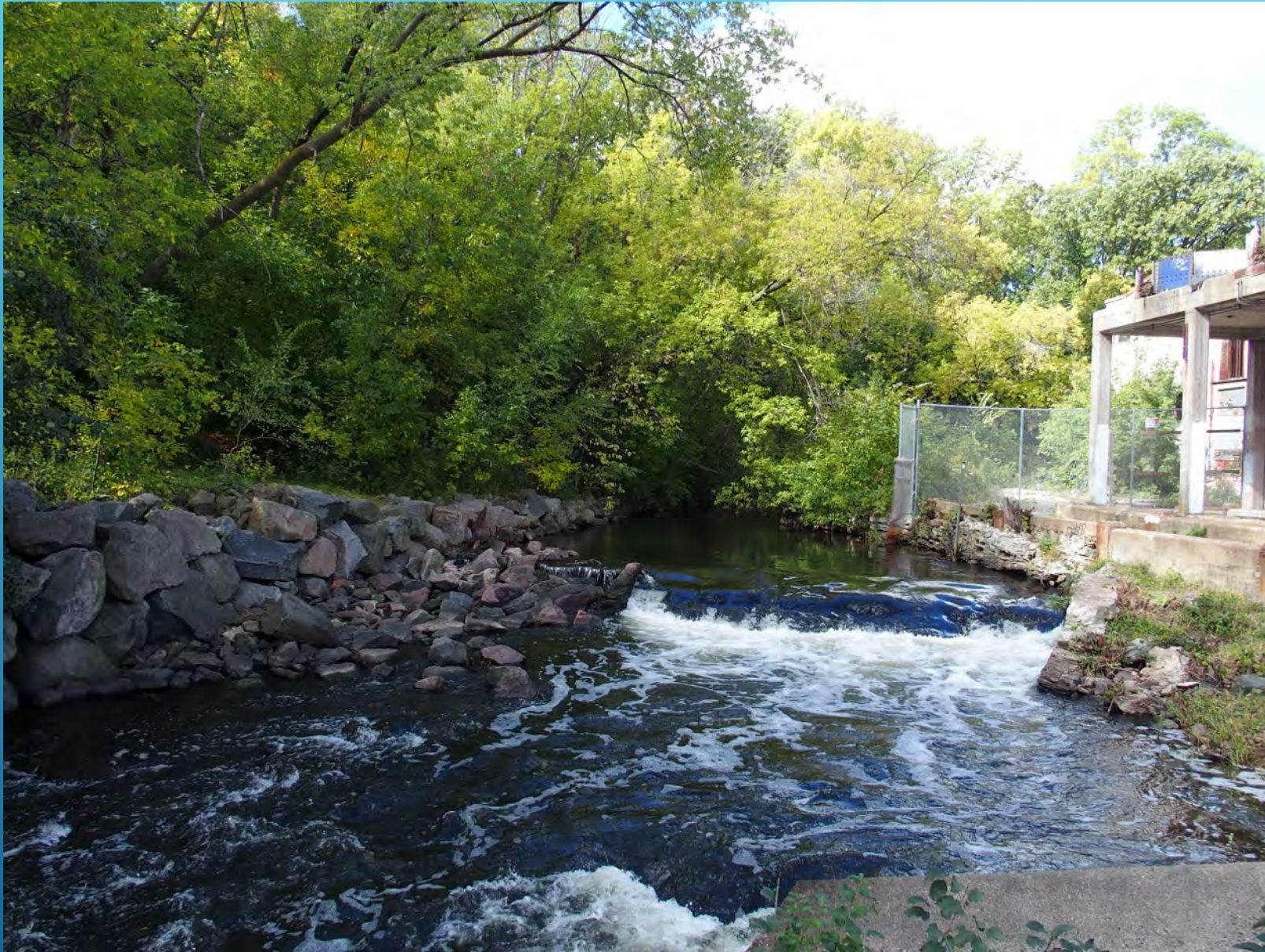
Bassett Creek at Fruen Mill, Minneapolis
