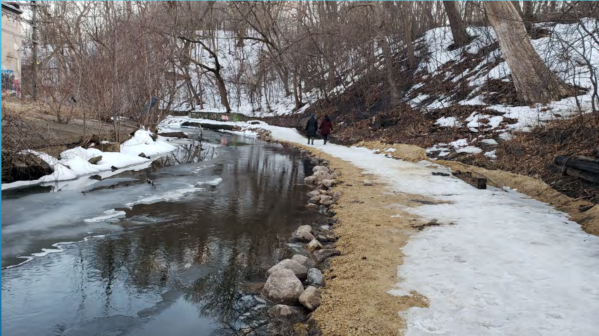
Bassett Creek Stabilization Project, Fruen Mill
