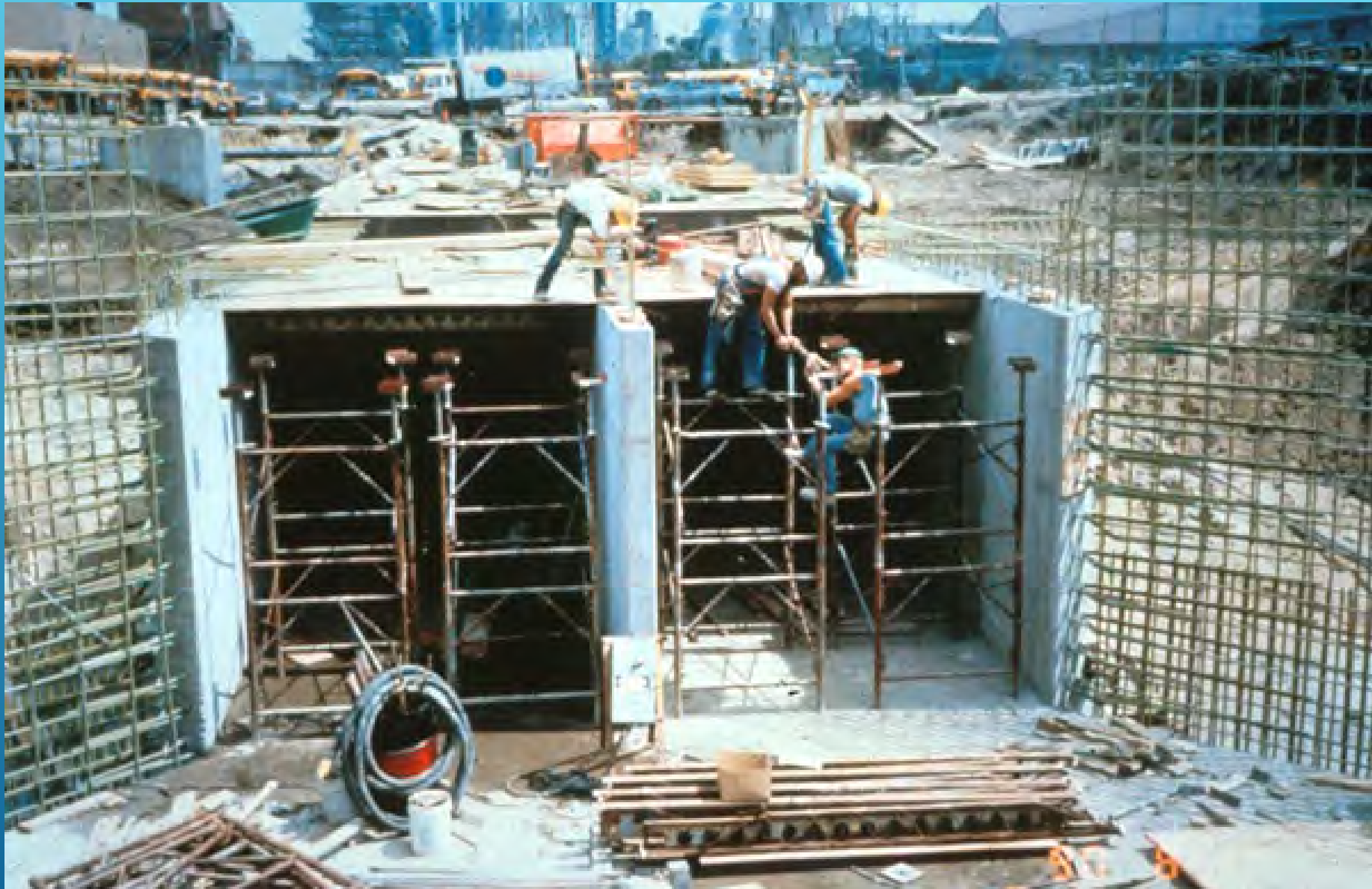
Bassett Creek Tunnel Double Box Culvert Construction 1990
