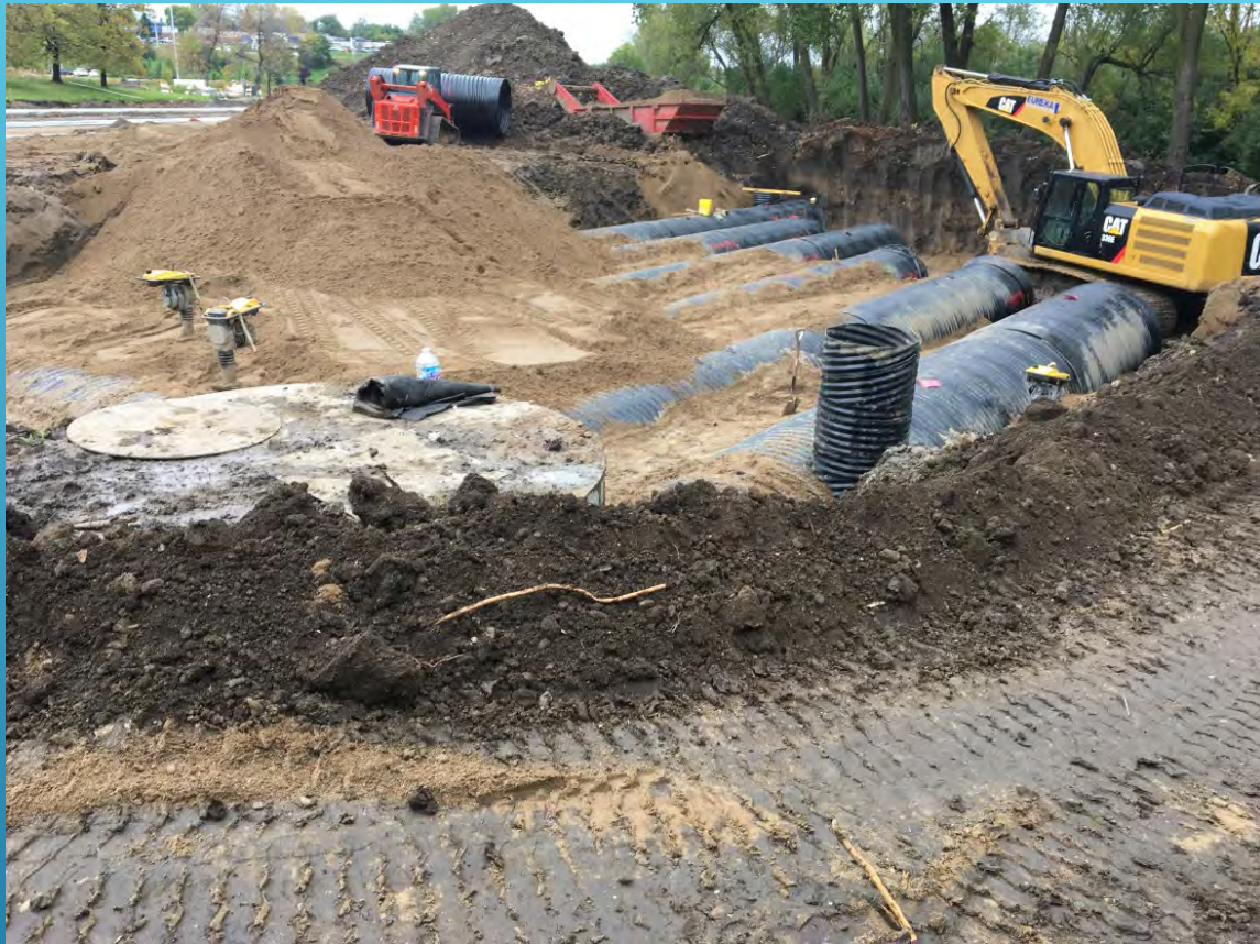
During and after construction
