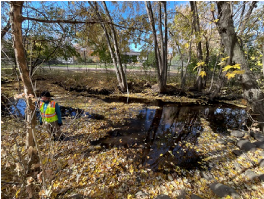
Photo 38: Site 3i. Left bank of station 53+50.
