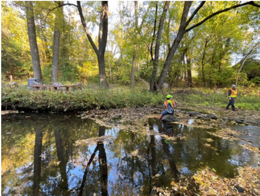
Photo 18: Site 2f. Left bank undercutting at station 23+10.
