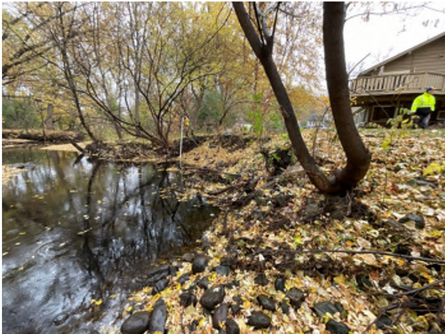
Photo 26: Site 2m. Soil exposure and deposition at the right bank of station 35+60 (facing downstream).
