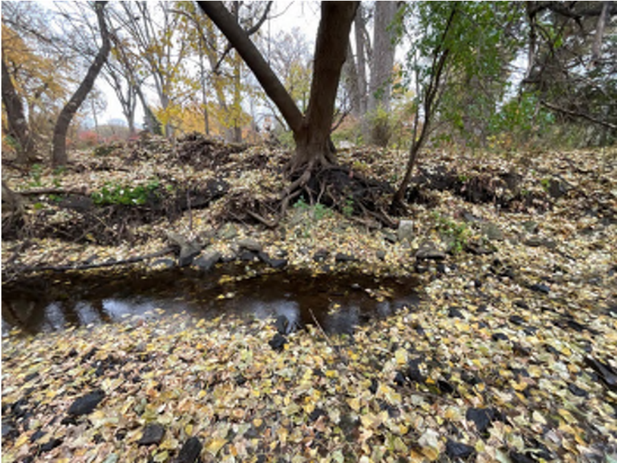
Photo 24: Site 2k. Undercutting at the right bank of station 32+25.
