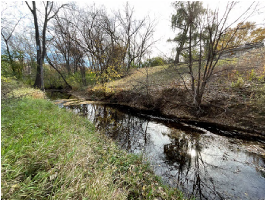
Photo 42: Site 4b. Right bank of downstream section at station 60+00.
