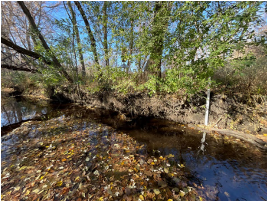
Photo 32: Site 3d. Upstream section of the left bank of station 47+50.
