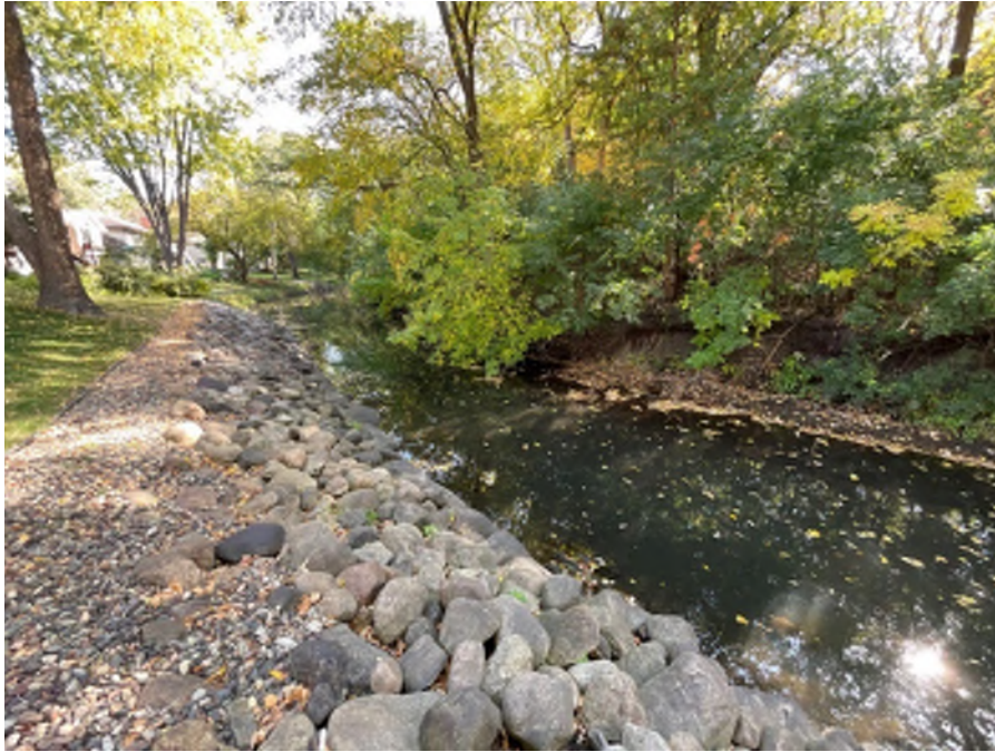
Photo 3: Site 1b. Downstream section at the right bank of station 4+50.
