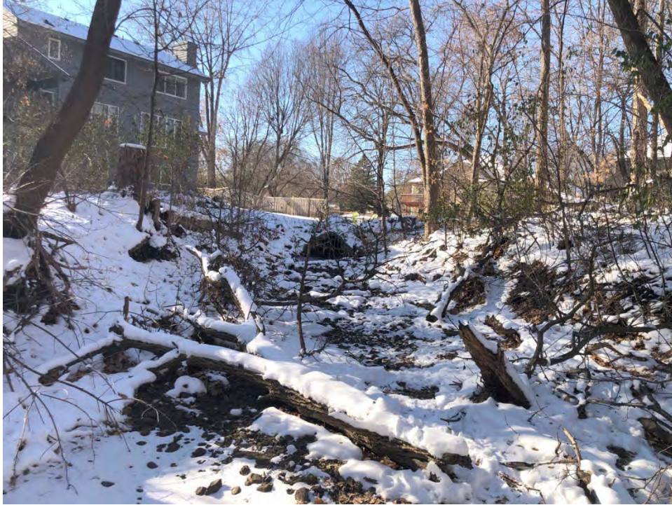
Figure 3-2 Upstream Section with Channel Debris and Bank Erosion (Reach 1)
