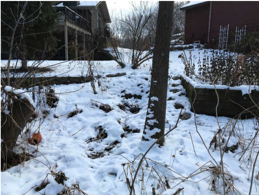
Figure A- 16 Upstream end of southeast stormwater side-channel.
