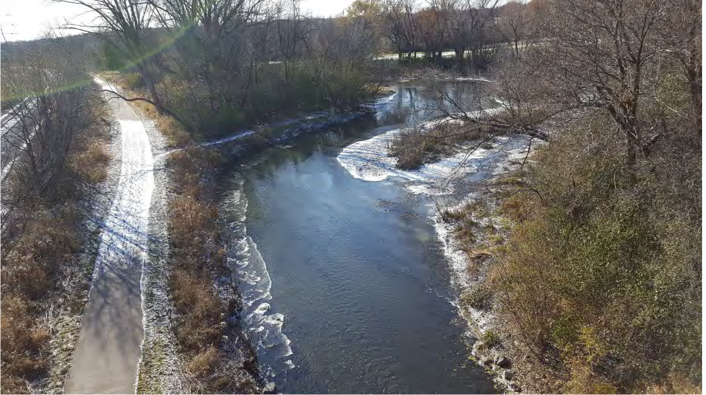
Photo 1: Lagoon D before construction, November 22, 2019
